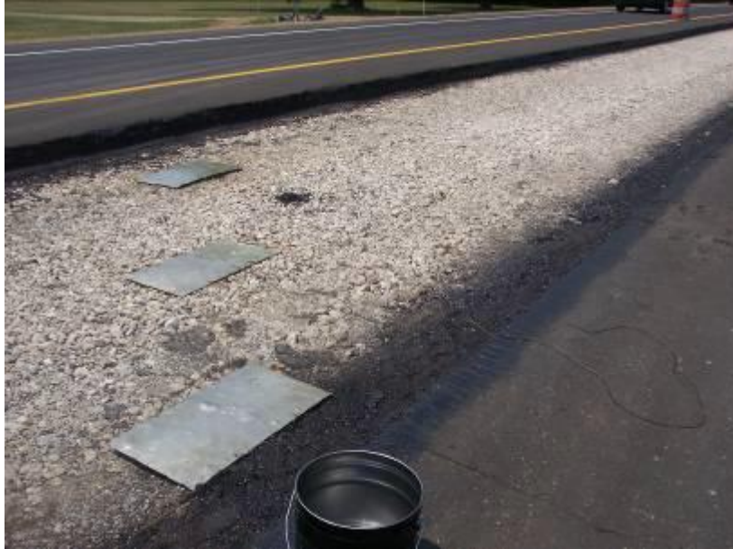
Figure 76 Plates randomly placed under AC mat
