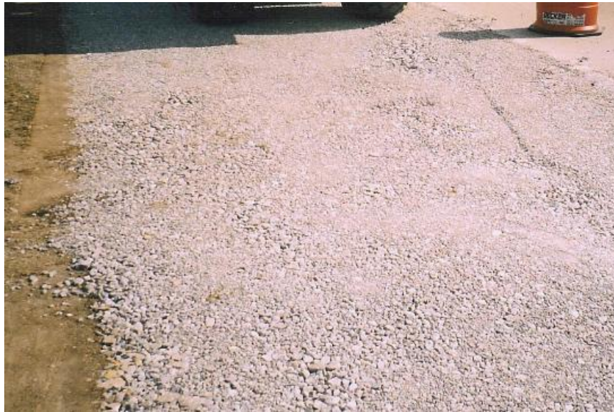
Figure 50. Surface created by drum rolling (from Ceylan et al. 2005)
