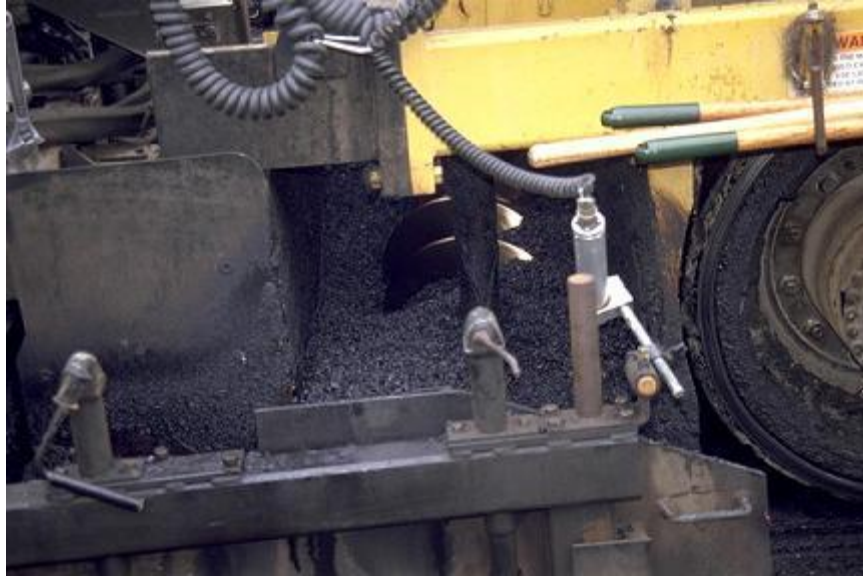
Figure 67. AC head in auger (Mahoney, Pavement interactive.com)
