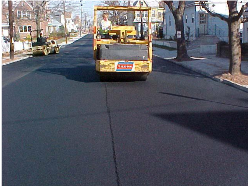
Figure 72 Rolling of hot mat for joint compaction (Benson and Scherocman 2006)
