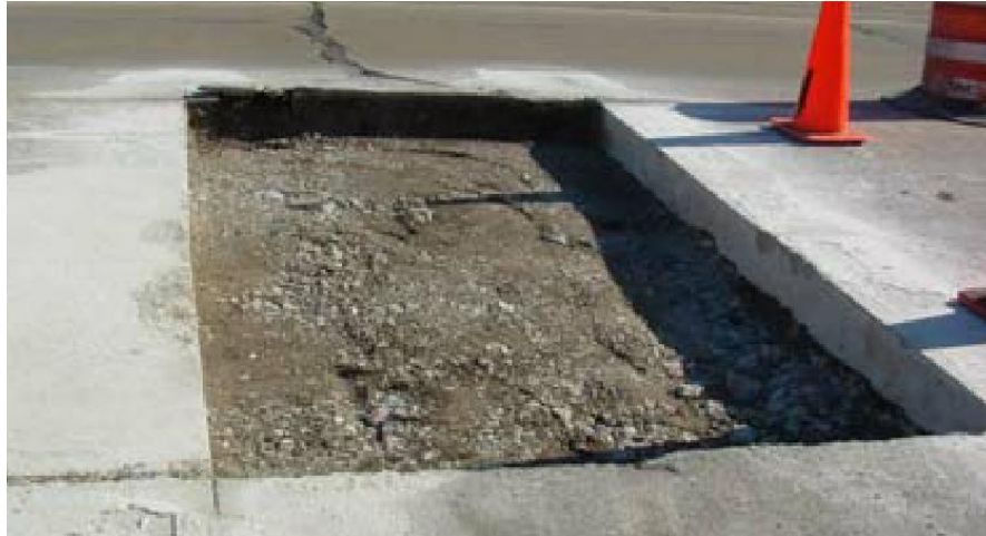
Figure 36. An undoweled full-depth repair in progress, the damaged concrete has been removed and the area has been cleaned. (Wen et al. 2005)
