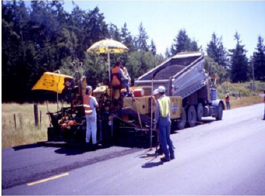
Figure 66. End dump of AC into paver hopper (Mahoney, Pavement Interactive.com)
