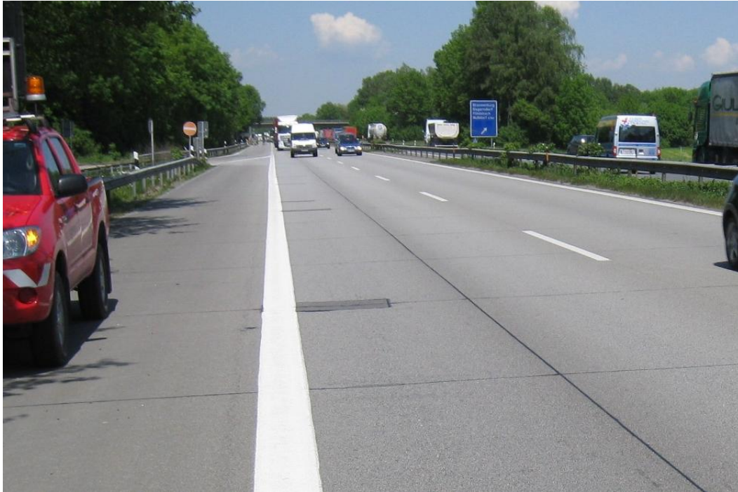
Figure 78. SMA over PCC along A93 in Germany, rectangular patch repair visible next to red traffic diversion truck (from Tompkins et al. 2010)
