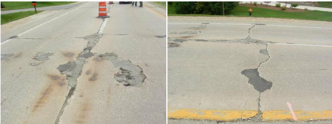
Figure 31. Spalled cracks which were previously patched; these areas will require either full- or partial-depth repair prior to placement of an AC overlay (Wen et al. 2005)
