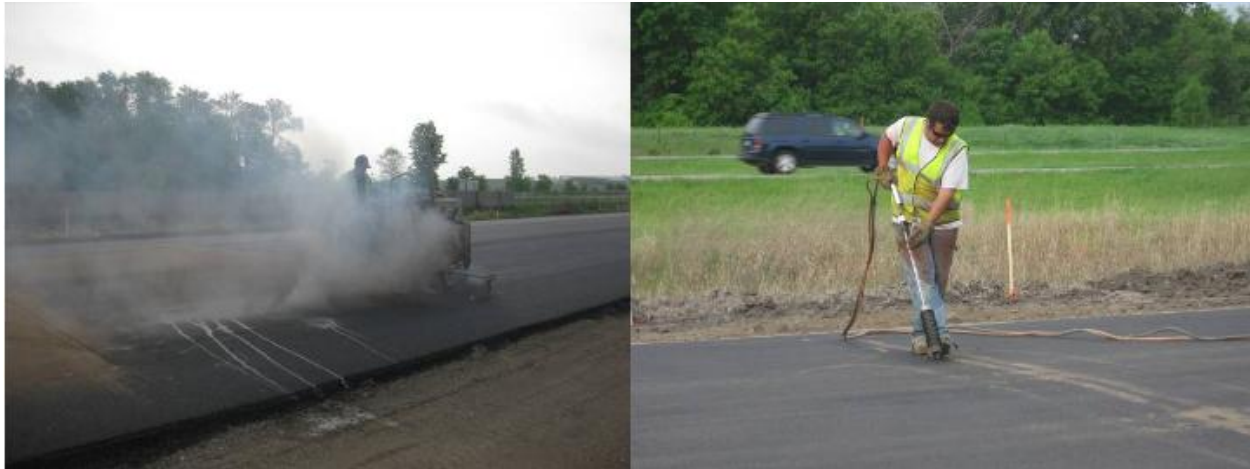
Figure 73. Sawing joints in the AC layer which correspond to the joints in the underlying PCC layer (left) and sealing the newly sawed joints (from Rao et al. 2011)
