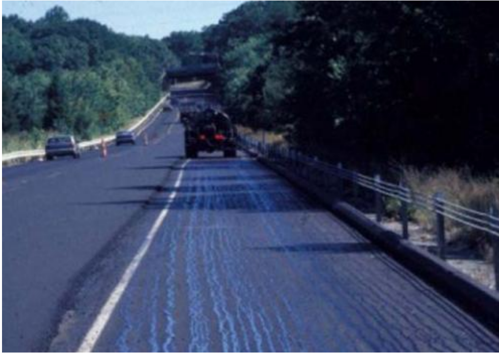
Figure 60. Improperly applied tack coat which leaves zebra stripes (from Mohammad et al. 2012).
