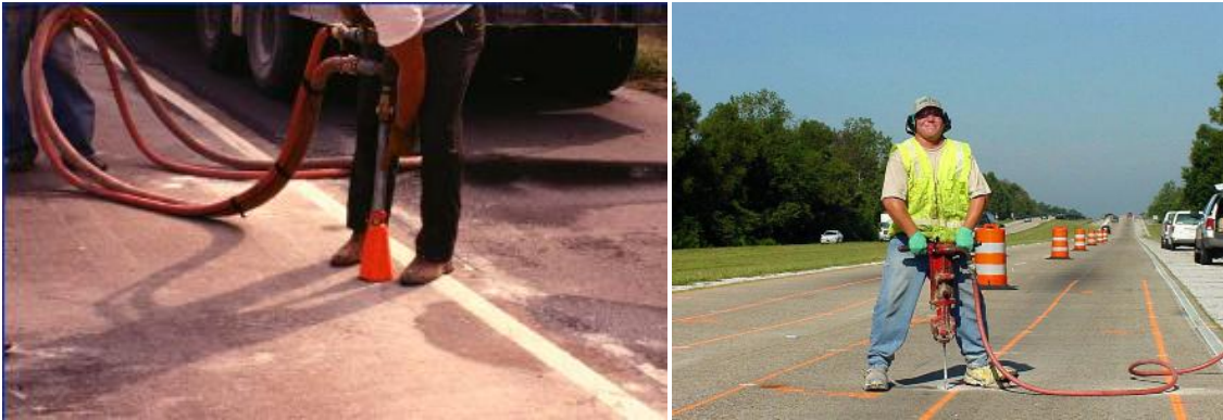
Figure 27. At left, slab stabilization; at right, removal of material for slab jacking (from Smith 2009)
