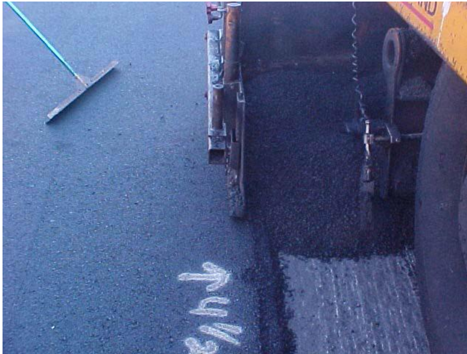
Figure 71 Proper overlap of hot mat onto cold mat (Benson and Scherocman 2006)
