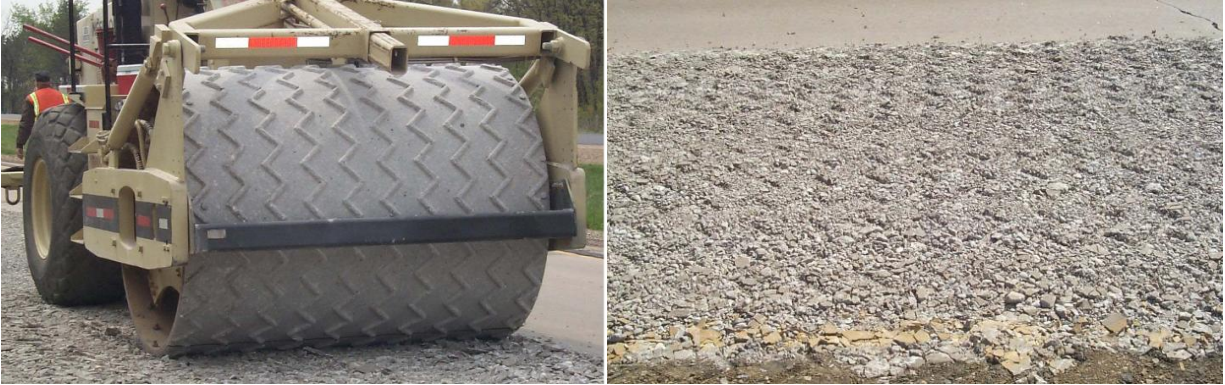
Figure 49. Grid the rubblized pavement (left), and the surface created by grid rolling (from Ceylan et al. 2005)
