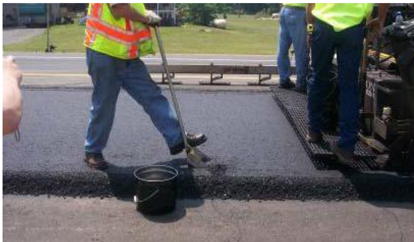
Figure 77 Shoveling material from above plates
