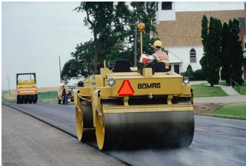
Figure 70 Proper rolling of free edge (Benson and Scherocman 2006)
