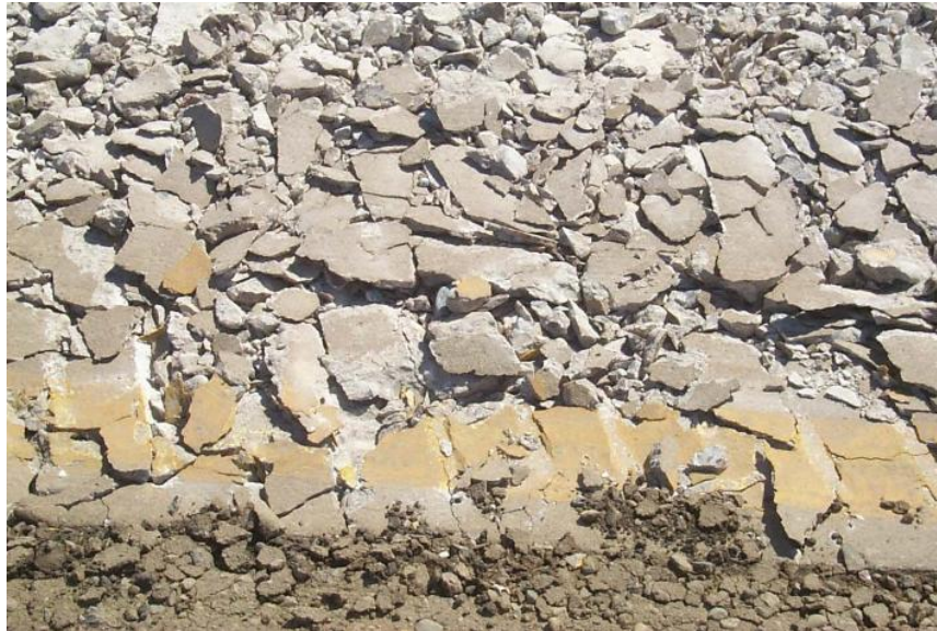
Figure 48. Existing concrete pavement after being rubblized using MHB method (from Ceylan et al. 2005)
