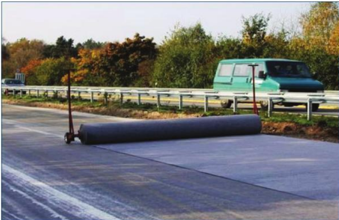
Figure 64. Placement of a geosynthetic interlayer fabric (from Harrington et al. 2008)
