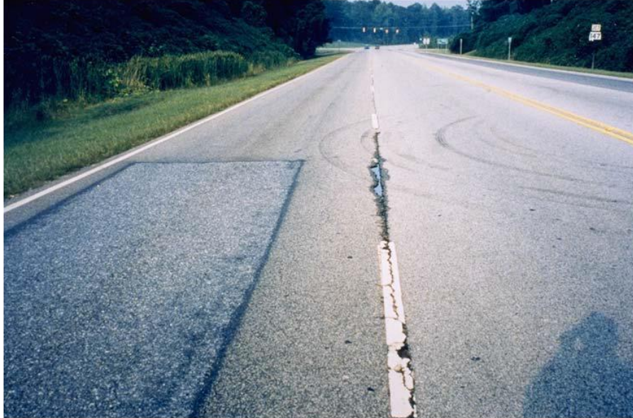
Figure 69 Raveled longitudinal joint (Brown, 2006)
