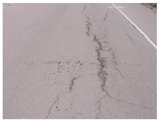
Photograph 3. Picture of what appears to be moisture at the surface of cracks on section 35\_0802.
