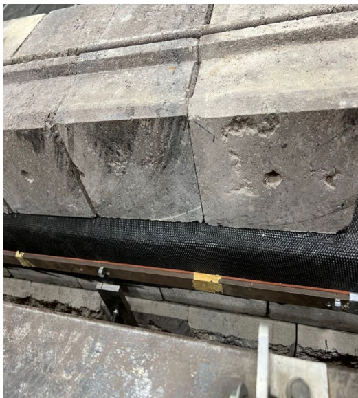
Figure 2.9 Geotextile installation between facing blocks
