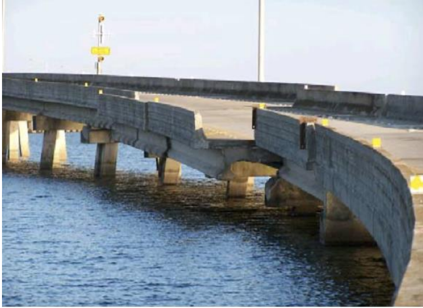
Figure 5: Displaced Segments on I-10 – U.S. 90 Ramp in Mobile Bay
