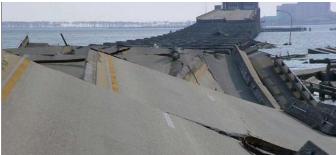
Figure 7: Damage to the Biloxi-Ocean Springs Bridge (from Ocean Springs, Mississippi)
