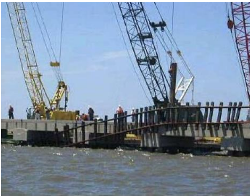
Figure 6: Cranes Used to Right the Rails on the Norfolk Southern Bridge
