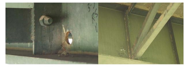
Figure A.13: (a) Close up of web gap region of bridge in a region of positive moment and (b) Cross-frame-to-web connection
