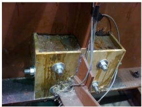
Figure B.39: Interior view of the girder a) Prior to casting the West System™ two-part epoxy. b) View of the cured composite blocks
