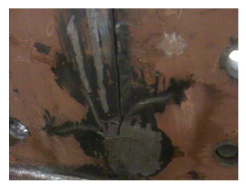
Figure B.66: Existing cracks on exterior face of the girder's web
