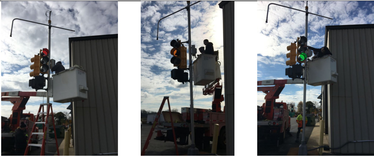
Figure 5 Field installation and setup of the onsite testing at the test site of Michigan in front of the signal shop, with the aid of the signal crew of Michigan DOT. A tunnel visor was installed with hook for mounting the cable camera on each signal module. The signals are facing north.
