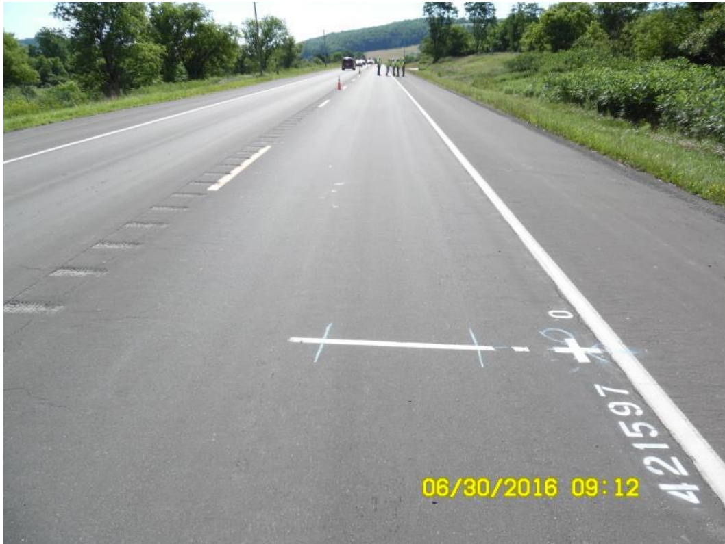
Photograph 1. LTPP Section 42_1597 at Station 0+00 looking eastbound in 2016.
