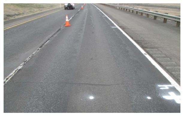
Figure 18. Condition of the pavement at station 400 prior to coring. The white dots are FWD test locations.
