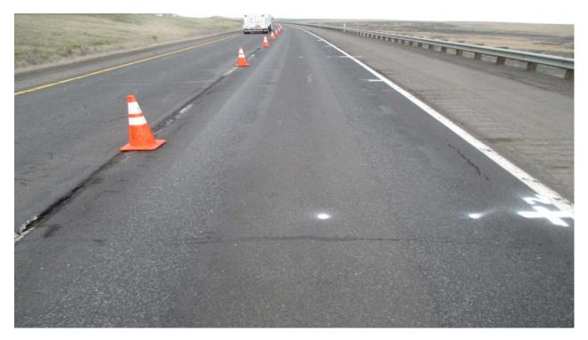
Figure 12. Image of station 200 prior to coring in 2019. The white dot paint marks are locations for FWD measurements.
