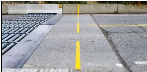
One of the electrified guards and steel grounding plate (left) and the 2 m yellow line from the electrified barrier (middle) (Photo Parks Canada).
