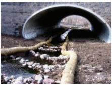
FIGURE 30. THIS CULVERT ON US 93 NORTH WAS ENLARGED TO ACCOMMODATE WILDLIFE PASSAGE IN ADDITION TO WATER FLOW.
