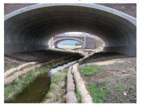
FIGURE 23. US 93 CONSPAN ARCH WILDLIFE CROSSING BRIDGES. PHOTO CREDIT. P. BASTING.
