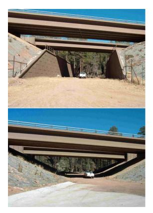
FIGURE 55. ARIZONA STATE ROUTE 260 WILDLIFE CROSSING BRIDGES WITH AND WITHOUT RETAINING WALLS. PHOTO CREDIT: T. BRENNAN.
