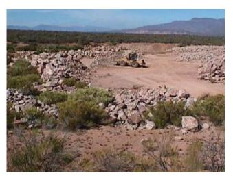
FIGURE 36. CONTRACTOR SORTING MATERIAL FOR RIP RAP AND AGGREGATE PRODUCTION IN ARIZONA, STATE ROUTE 188, AND ON THE TONTO NATIONAL FOREST. PHOTO CREDIT: T. BRENNAN.
