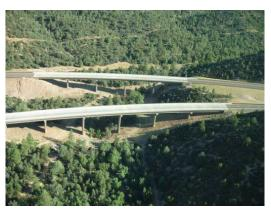
FIGURE 53. TWO OF THE LARGE WILDLIFE CROSSING BRIDGES ON STATE ROAD 260, PAYSON, ARIZONA. PHOTO CREDIT: T. BRENNAN.
