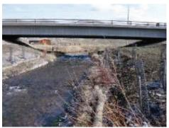
FIGURE 31. THIS BRIDGE ON US 93 IN THE BITTERROOT VALLEY WAS LENGTHENED TO ACCOMMODATE WILDLIFE PASSAGE. PHOTO CREDITS: L. FRAZIER.
