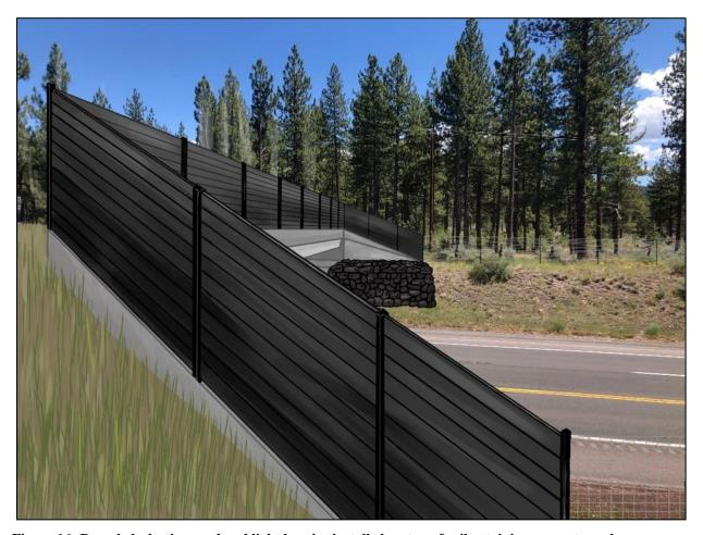
Figure 16: Recycled-plastic sound and light barrier installed on top of soil-retaining concrete curb.
