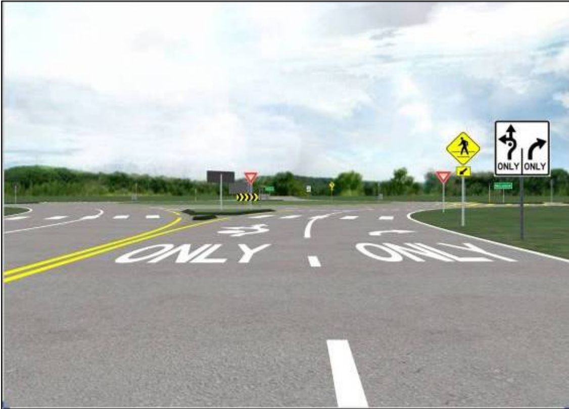
Figure 4: Example of Fishhook Arrows with Words Scheme (FAW) – Type D Lane Restrictions
