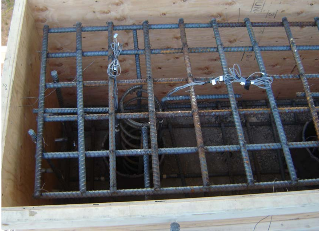
Figure 3-14 Photograph of Pile Cap 1 reinforcing.
