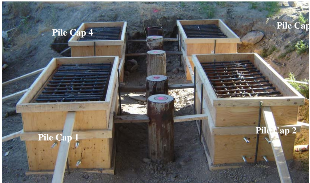
Figure 3-4 Photograph of the pile cap reinforcing and forms prior to concrete placement as the South Temple, Salt Lake City Test Site.
