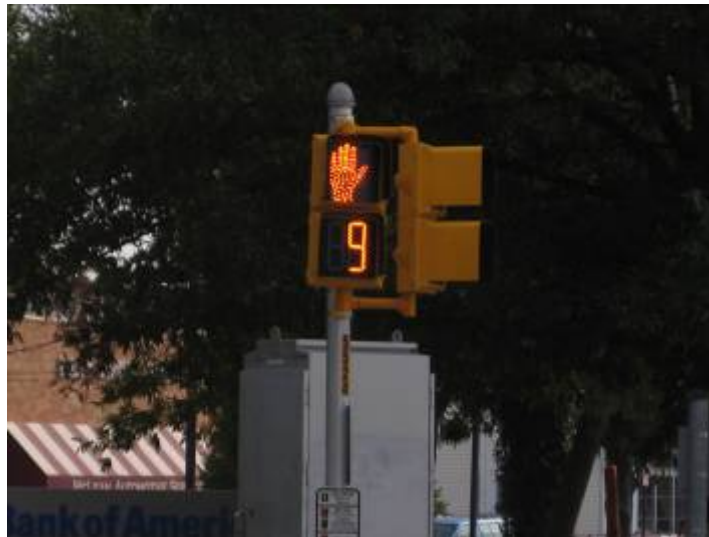
Figure 1: Example of a Countdown Pedestrian Crossing Signal Head in McLean, Virginia.
