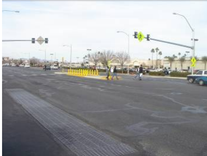
Figure 3: Possible Site for Installation of Enlarged Pedestrian Countdown Signals in Las Vegas, NV.
