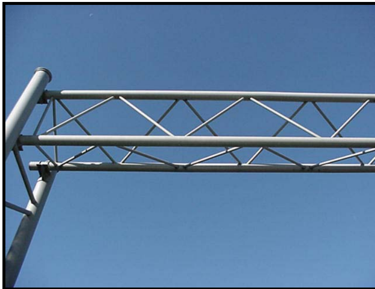
Figure 1. Tri-truss aluminum overhead sign support structure
