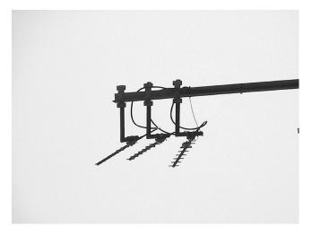
FIGURE 4 AVI antenna configuration.
