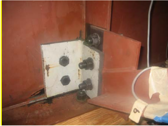
Fig 6. View of angle retrofit in bottom web gap; connection is made between the web and connection stiffener
