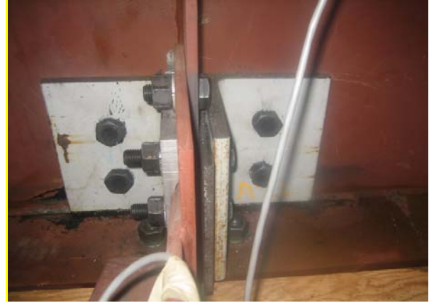
Fig 7. Alternate view of angle retrofit in bottom web gap; connection is made between the web and connection stiffener
