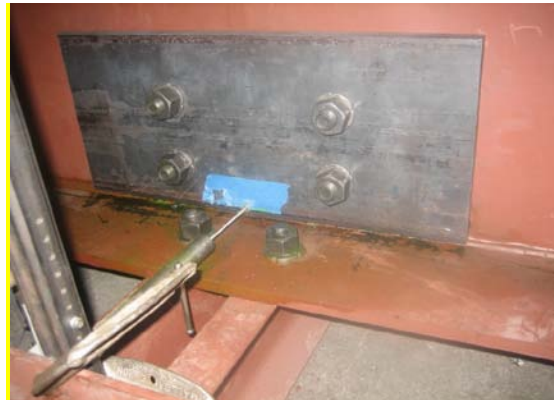
Fig 8. Fascia view of angle retrofit in bottom web gap; steel back plate is applied on fascia side of girder to aid in load transfer around the web gap region.
