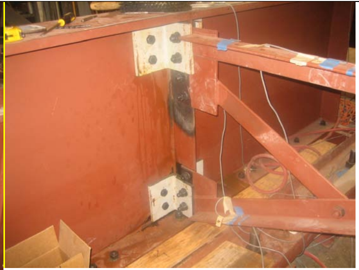
Fig 10. Interior view of girder after angle retrofit has been applied to both the top and bottom web gap
