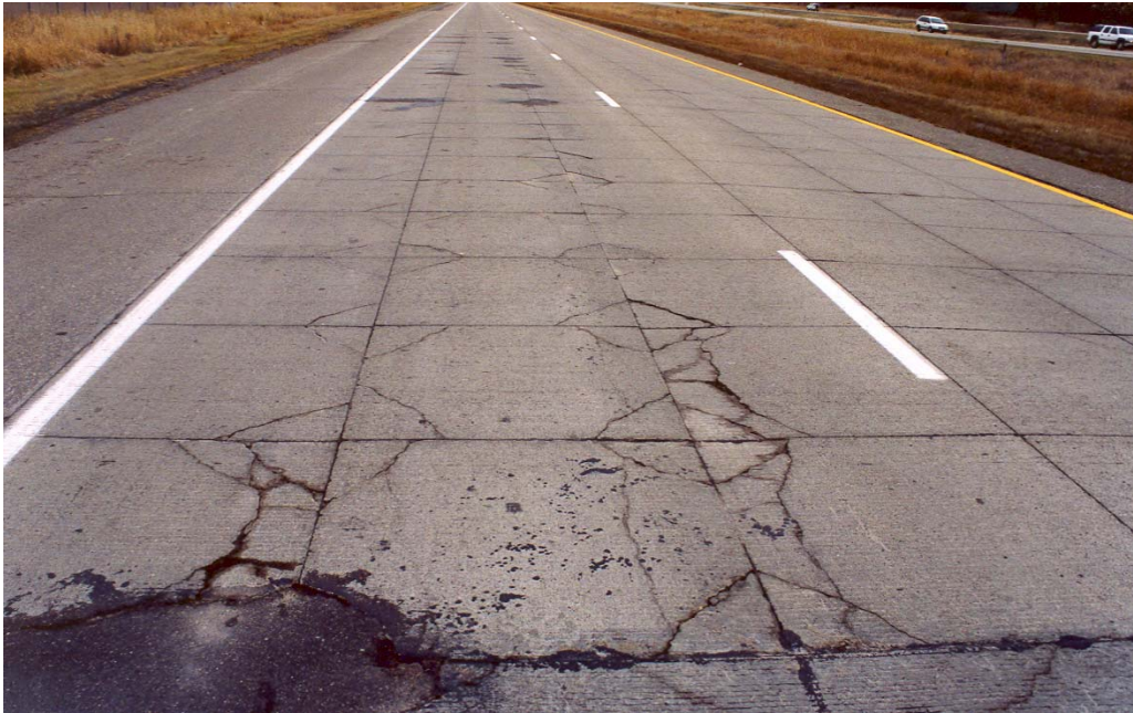
Photo 1. Major distress in ultra-thin whitetopping at the MnROAD project, observed before the forensic evaluation in 2004.
