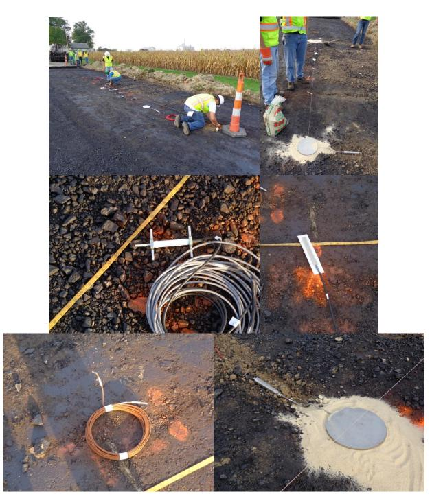
Figure C-3. Instrumentation at the bottom of DGAB in section A
