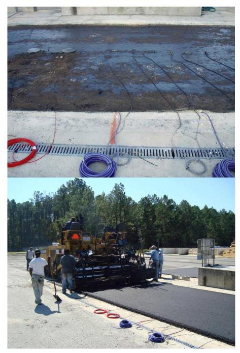
Figure B-1. Sensors before and after paving Florida DOT
