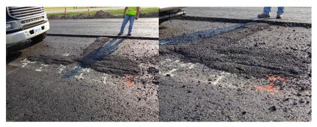
FigureC-9. Possible misalignment of sensors after truck passes
