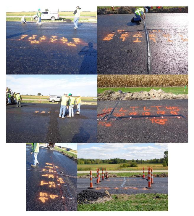
FigureC-11. Instrumentation at the bottom of the intermediate layer
