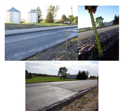
FigureC-13. Milling and fill of ATB in Section A
