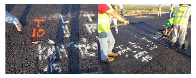
FigureC-8. 45° strain gauge 1 ft apart from adjacent sensors
