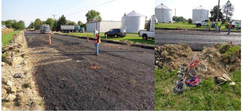
Figure C-4. Installation of sensor at the bottom of the FRL in Section A
