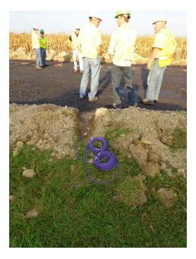
Figure C-2. Geokon pressure cells on top of the subgrade
