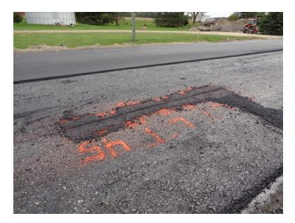
FigureC-14. Truck ran over sensor in Section A
