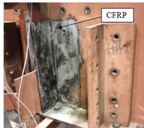
Figure 7. View of the steel-CFRP sandwich retrofit applied to Specimen 3 (interior face of girder; right side of connection stiffener) – steel angle has been removed from the CFRP in this view
