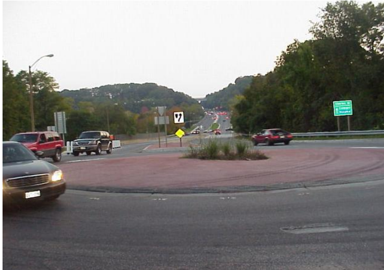
FIGURE 5.10 Roundabout North of Baltimore - Almost All Truck Apron
