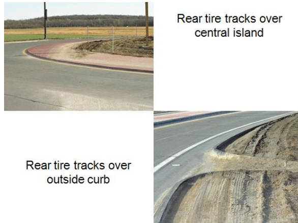
FIGURE 5.5 Truck Tracks Inside of Truck Apron and Center Island
