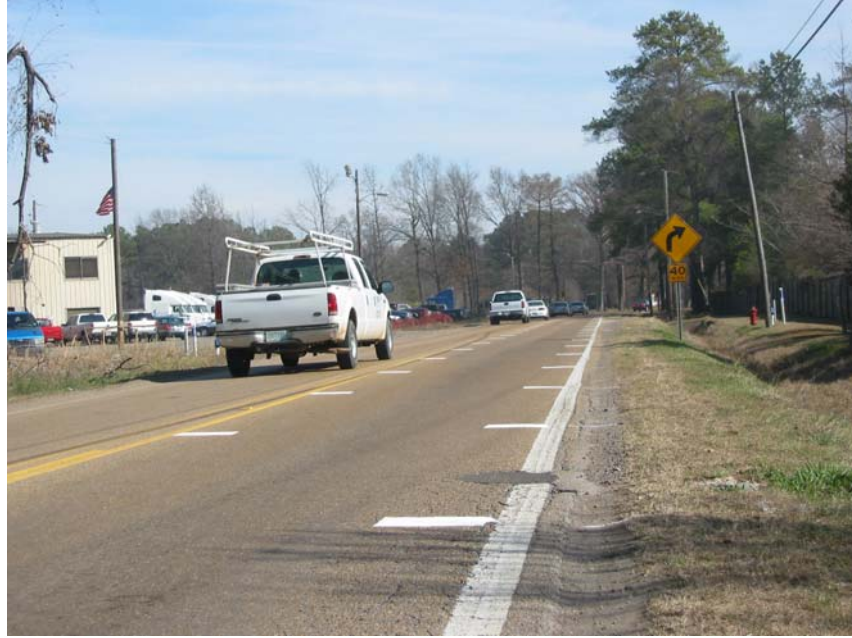
Figure 6: Peripheral Transverse Lines Treatment on MS 468 in Flowood, Mississippi
