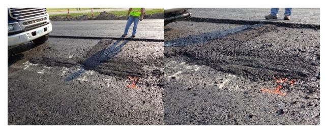
Figure 34. Possible misalignment of sensors after truck passes
