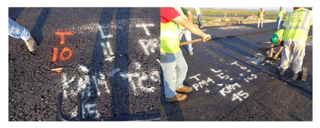
Figure 33. 45° strain gauge 1 ft apart from adjacent sensors
