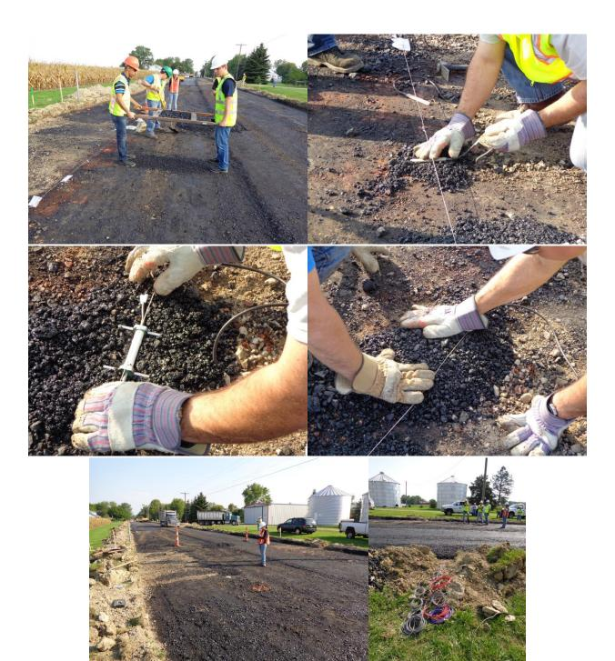
Figure 29. Installation of sensor at the bottom of the FRL in Section A
