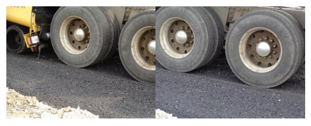
Figure 35. Rutting of FRL due to weak DGAB
