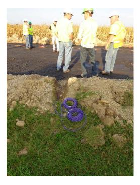
Figure 27. Geokon pressure cells on top of the subgrade
