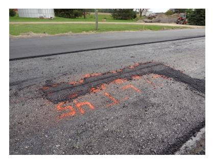
Figure 39. Truck ran over sensor in Section A
