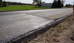
Figure 38. Milling and fill of ATB in Section A
