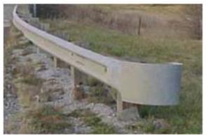
Figure 1-1 Breakaway Cable Terminal (BCT)
