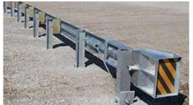
Figure 4-3 Flared Energy Absorbing Terminal (FLEAT<sup>TM</sup>)
