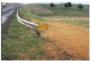
Figure 1-2 Modified Eccentric Loader Terminal (MELT)
