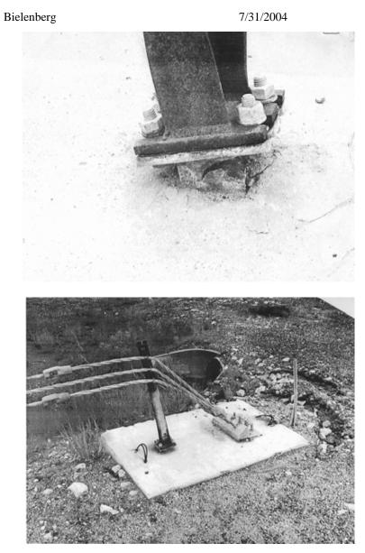
Figure 1. NY Cable Anchorage Damage
