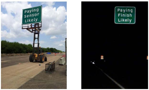
Figure 2. Overhead guide signs in the daytime and nighttime raised position.
