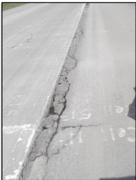
Figure C8.6. Alligator cracking Cell 13
