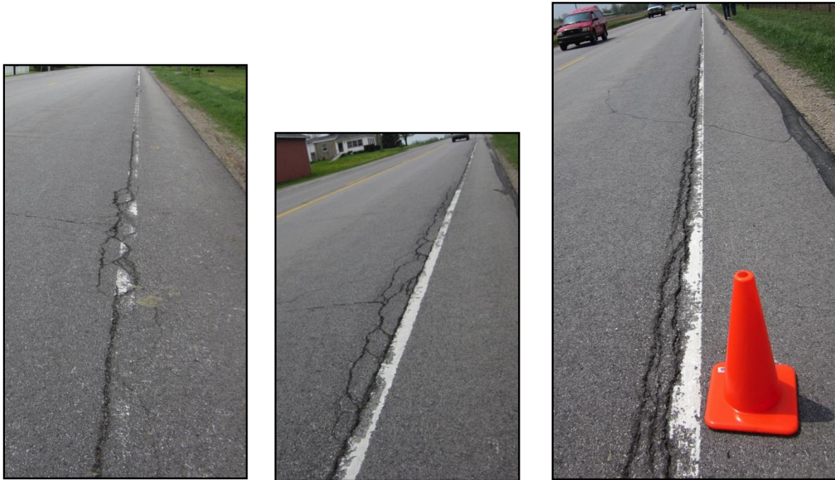
Figure D8.10. Longitudinal/block cracking near adjacent striping
