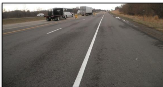
Figure C8.8. Medium raveling west transition
