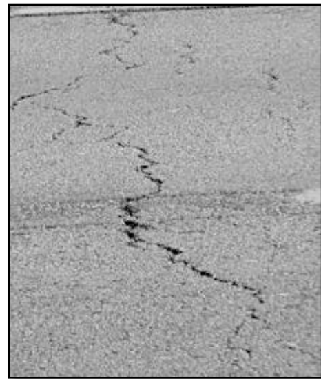
Figure A8.5. Medium severity TC (Control)
