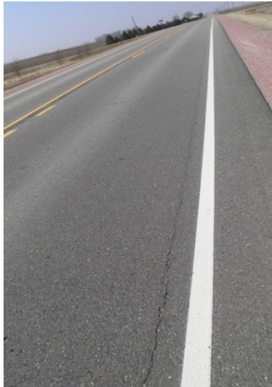
Figure B8.6. Longitudinal reflective cracking (HMA 0% RAS)
