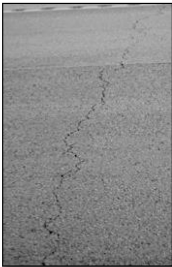
Figure A8.4. Low severity TC (Fine RAS)
