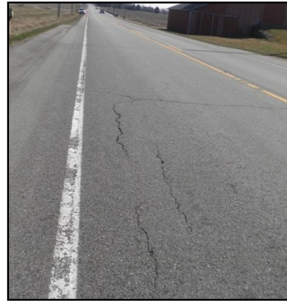
Figure D8.6. Fatigue cracking (HMA-RAP) Figure D8.7. Fatigue cracking (HMA-RAS)
