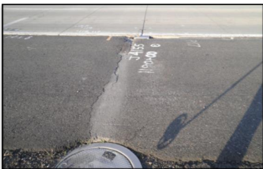
Figure C8.4. Transverse crack Cell 14
