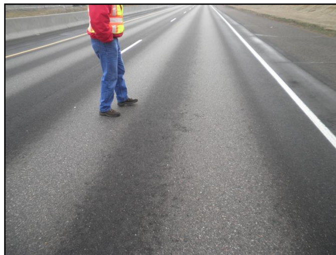
Figure F8.6. Low severity raveling (RAP)
