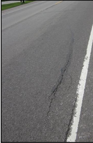
Figure D8.6. Fatigue cracking (HMA-RAP) Figure D8.7. Fatigue cracking (HMA-RAS)
