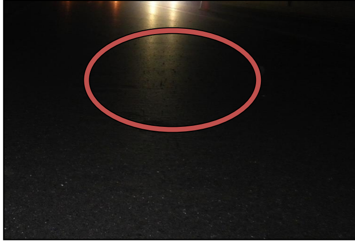
Figure F5.4. RAS tabs visible during paving
