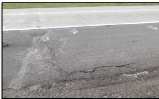
Figure C8.5. Block cracking Cell 13
