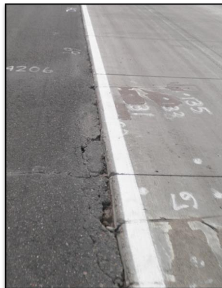
Figure C8.7. Alligator cracking Cell 14
