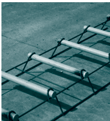
Figure 1. Typical dowel basket assembly
