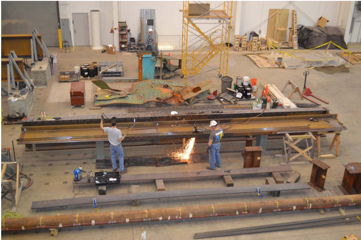
Figure 2: Specimen 30-1 fabrication – track torch cutting web plate to size
