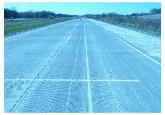
Figure A-9. Longitudinal tining downstream view.
