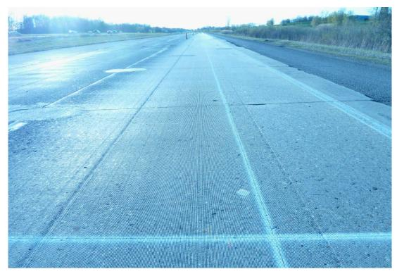
Figure A-11. Diamond grinding downstream view.
