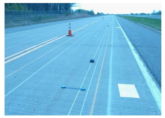
Figure A–7. Transverse tining downstream view.
