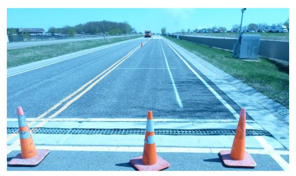
Figure A-5. Pervious hot mix asphalt downstream view.
