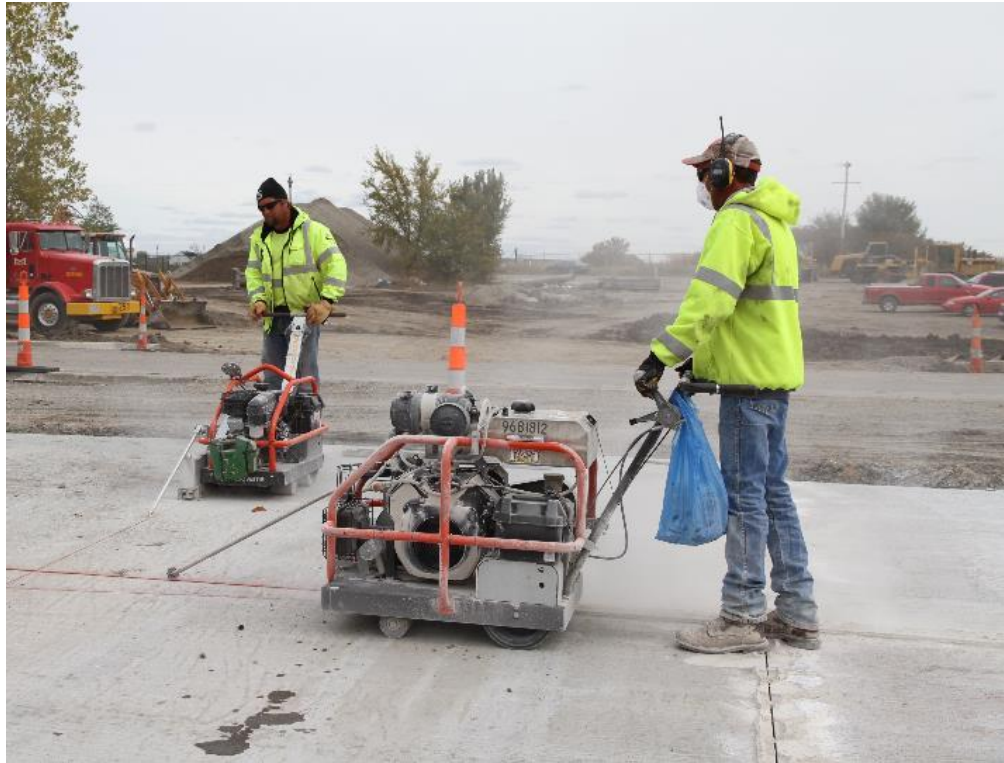
Figure 4. Use of early entry saws
