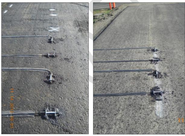
(a) Instruments on top of the recycled base (b) Strain gauges on top of the bottom lift of HMA Figure F-14. View of strain gauges and pressure cells installed on Section 671HC during construction.
