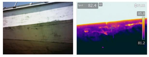
Figure 15: Standard and IR photos of bridge soffit delamination (Woodburn, Oregon)
