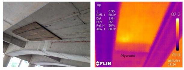
Figure 17: Standard and IR photos of bridge soffit (Waco, Texas)
