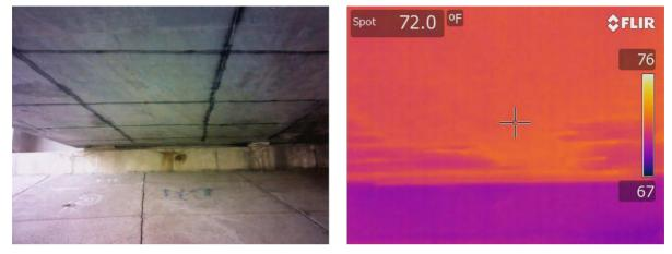
Figure 9: Standard and IR photos of bridge soffit delaminations (Duluth, Minnesota)
