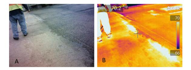
Figure 14: Delaminations along the edge of the deck
