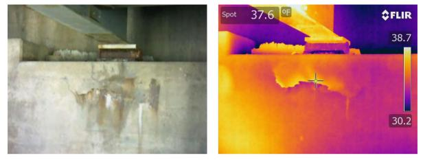
Figure 19: Standard and IR photos of bridge support delamination (Richland Center, Wisconsin)
