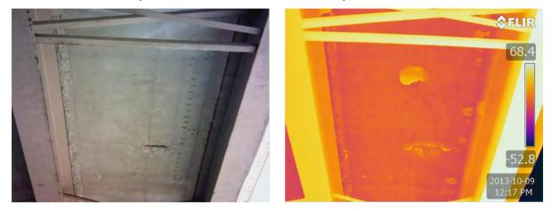
Figure 13: Standard and IR photos of bridge substructure delaminations (Harveysburg, Ohio)
