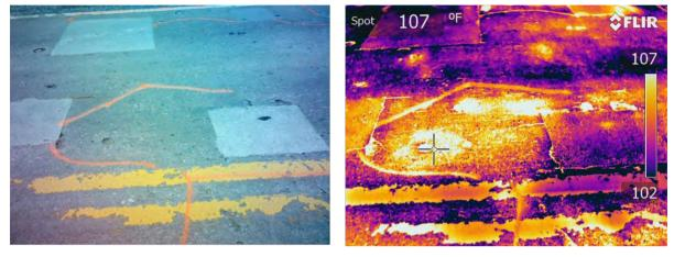
Figure 3: Standard and IR photos of bridge deck delamination (Barnesville, Georgia)
