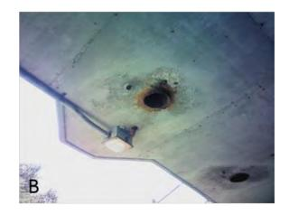
Figure 47: Afternoon infrared (A) and digital (B) images of a soffit delamination in
