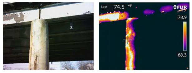
Figure 11: Standard and IR photos of bridge substructure delaminations (Albany, New York)
