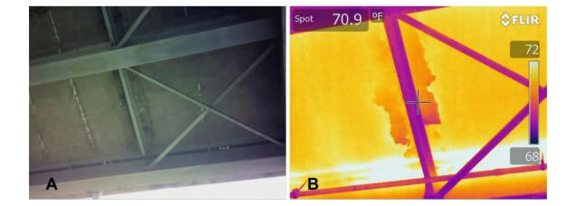
Figure 9: Delamination with some spalling by a cross brace in the soffit
