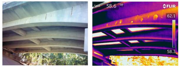
Figure 7: Standard and IR photos of bridge soffit delaminations (Mount Sterling, Kentucky)
