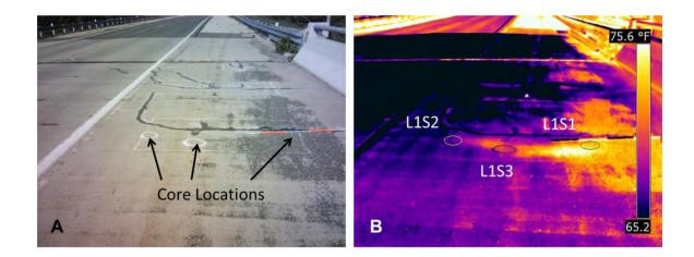
Figure 10: Cores at Location 1
