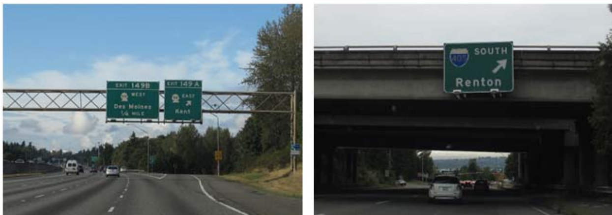
Figure 16 Example arrow placement on signs without EXIT ONLY panel (source: Scott Kuznicki).
