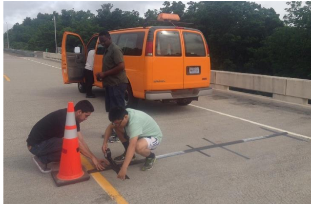
Figure 5 Installation of one-inch high electrical rubber cable cord
