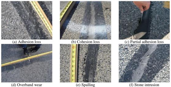
Figure 4. Commonly Observed Crack Sealant Distresses
