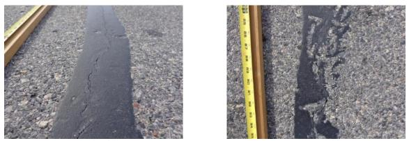
(a) Cohesive failure (b) Overband failure Figure 16. Common Failure Modes of Clean and Seal Treatment
