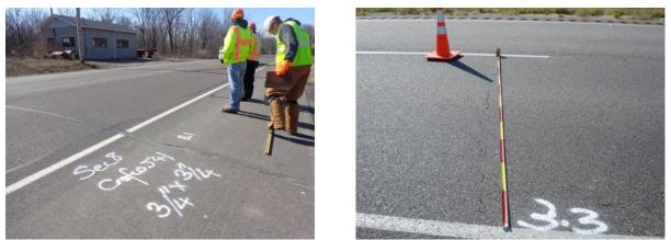
Figure 2. Initial Survey and Crack Numbering of a Test Section
