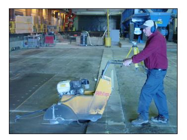
Figure 18. Dry saw cutting of the asphalt layer.
