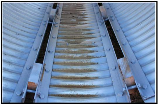
Figure A3: CMPs Invert Cut Detail
