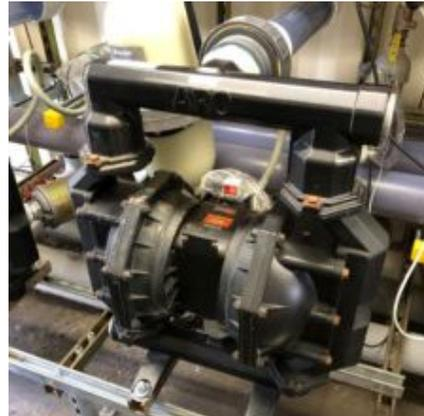
**Figure 4. Air-Operated Double Diaphragm Pump**
