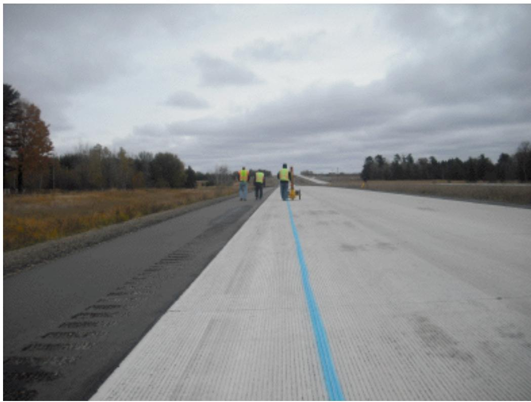
**Figure A-9. Longitudinal tining, downstream view, 2009.**
