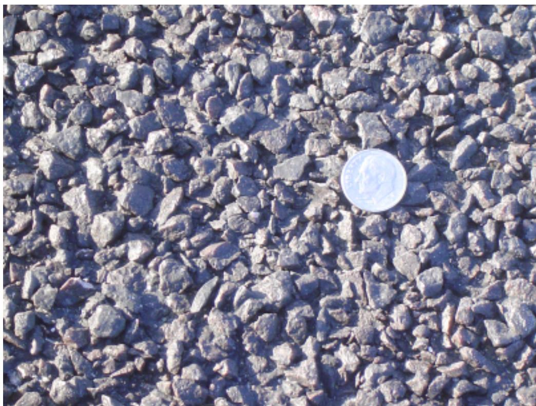
**Figure A–3. Chip seal, texture close-up, 2009.**
