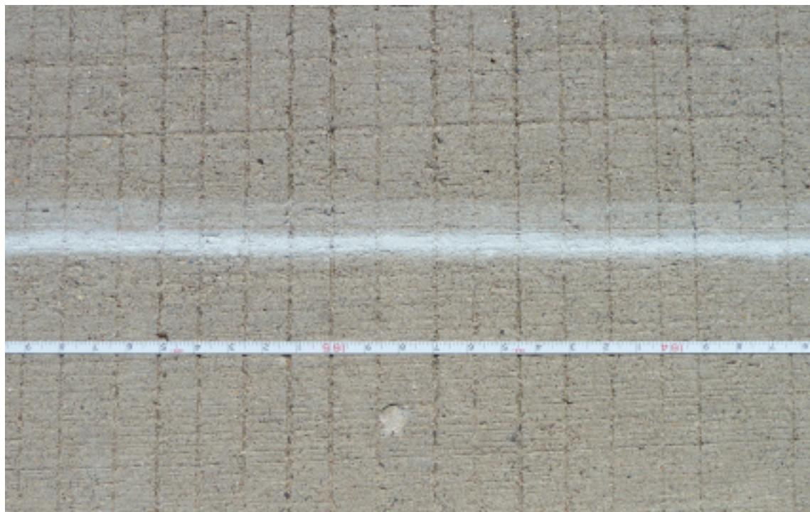
**Figure A–17. Transverse tining, with Benchmark Profiler guide tape, 2010.**
