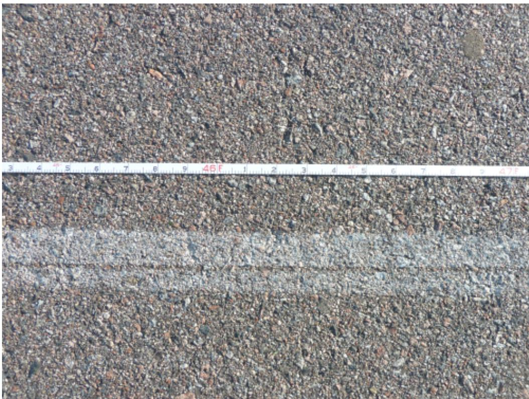
**Figure A–2. Dense graded asphalt, with Benchmark Profiler guide tape, 2010.**
