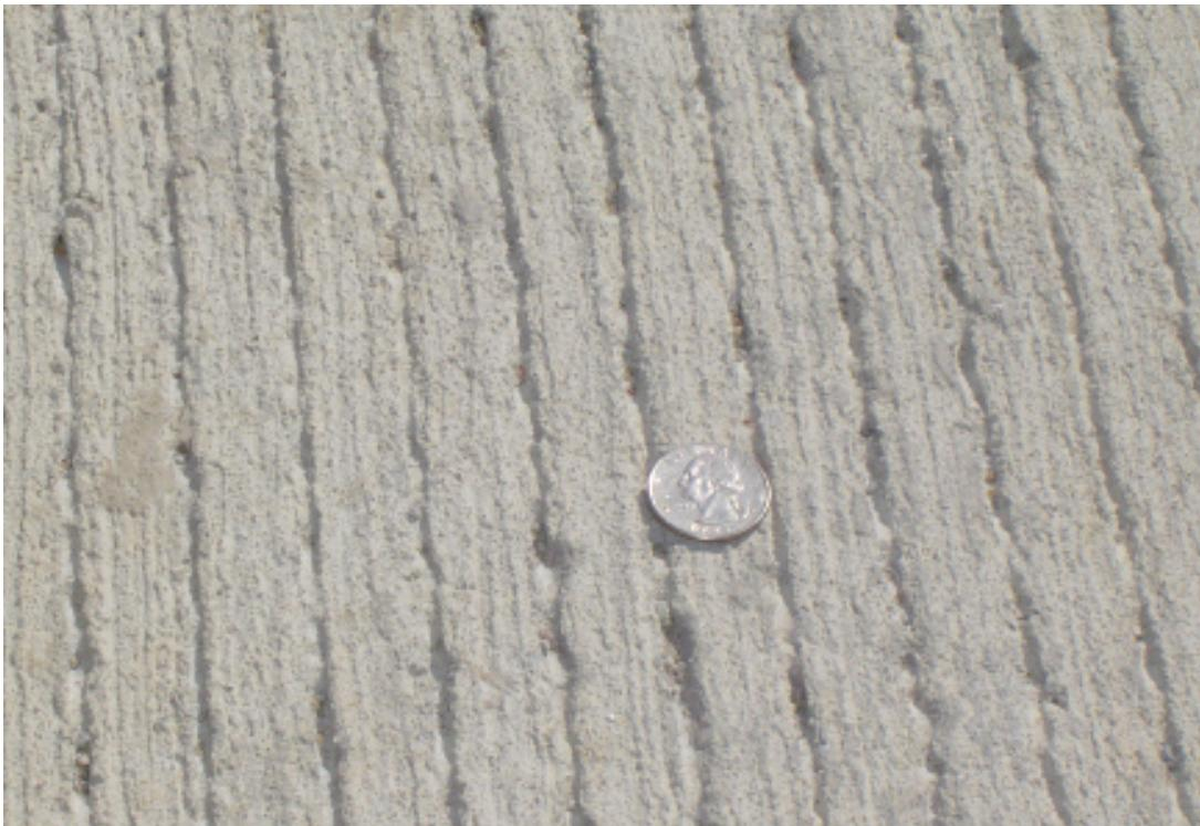
**Figure A–10. Longitudinal tining, texture close-up, 2009.**
