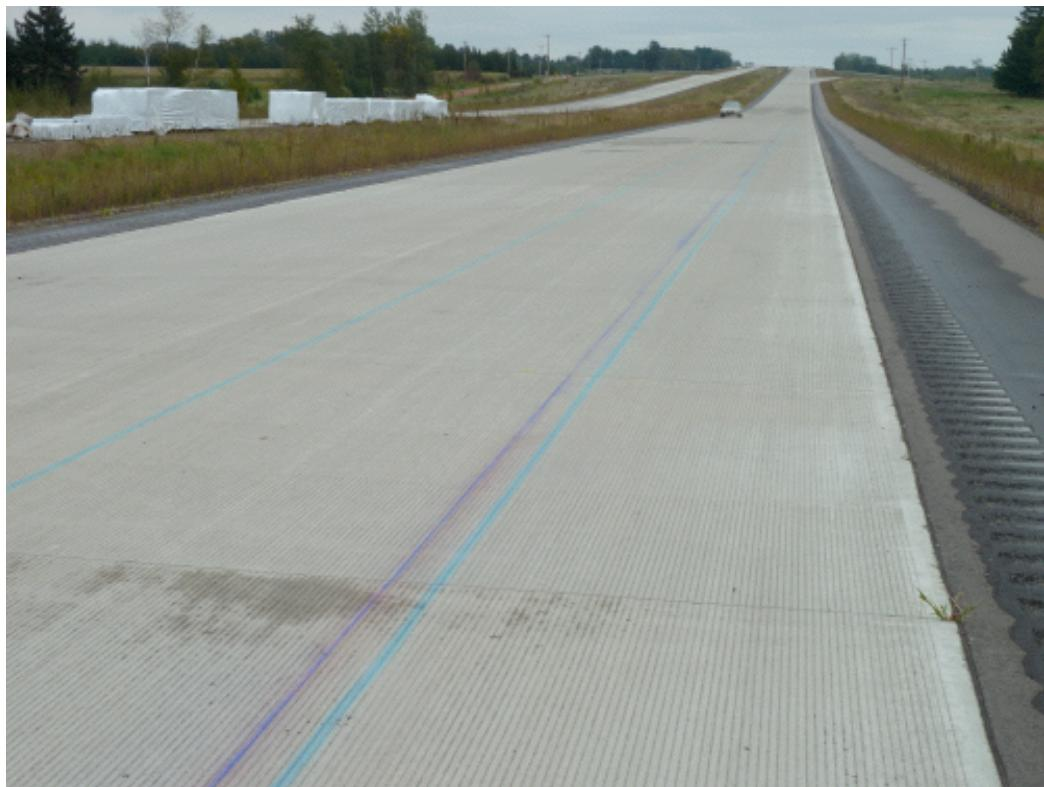
**Figure A–11. Longitudinal tining, downstream view with vendor chalk mark, 2010.**
