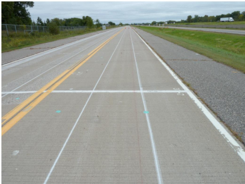
**Figure A–19 Transverse tining, downstream view, 2010.**
