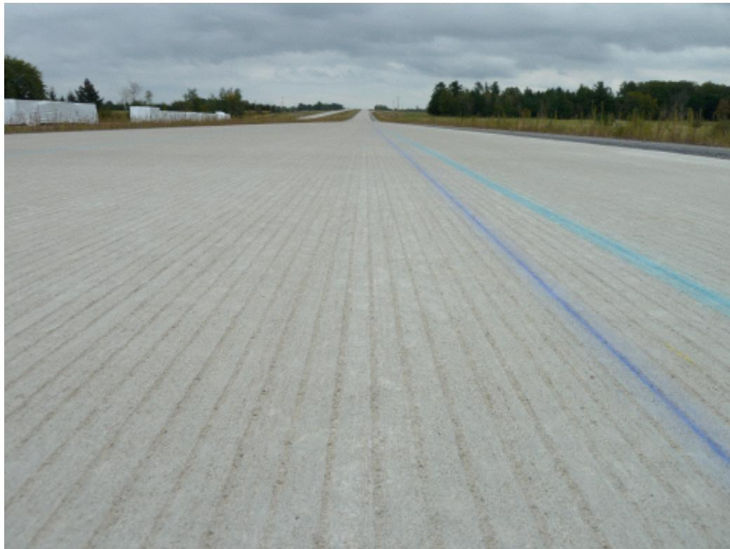
**Figure A–12. Longitudinal tining, texture close-up, 2010.**
