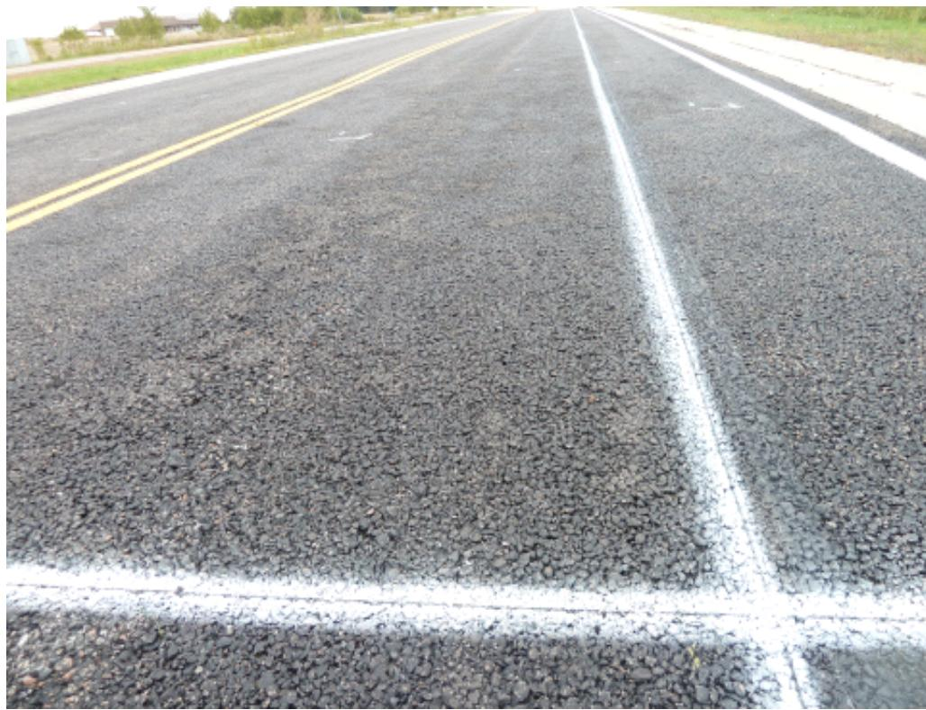
**Figure A–15.** Pervious hot mix asphalt, starting mark, 2010.
