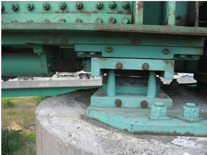
**Figure 171 Photo. Isolation in Illinois: Isolation Bearing (Poplar Street Complex – IL)**
