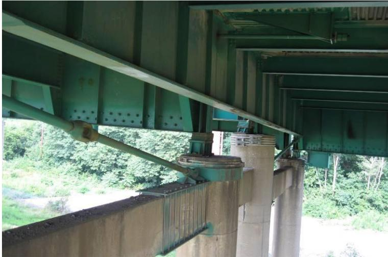
**Figure 154 Photo. Poplar Street Retrofits in Illinois: Bent Cap Retrofit, Longitudinal Restrainer Bars, and Transverse Restraint with Turnbuckles (Poplar Street Complex – IL)**
