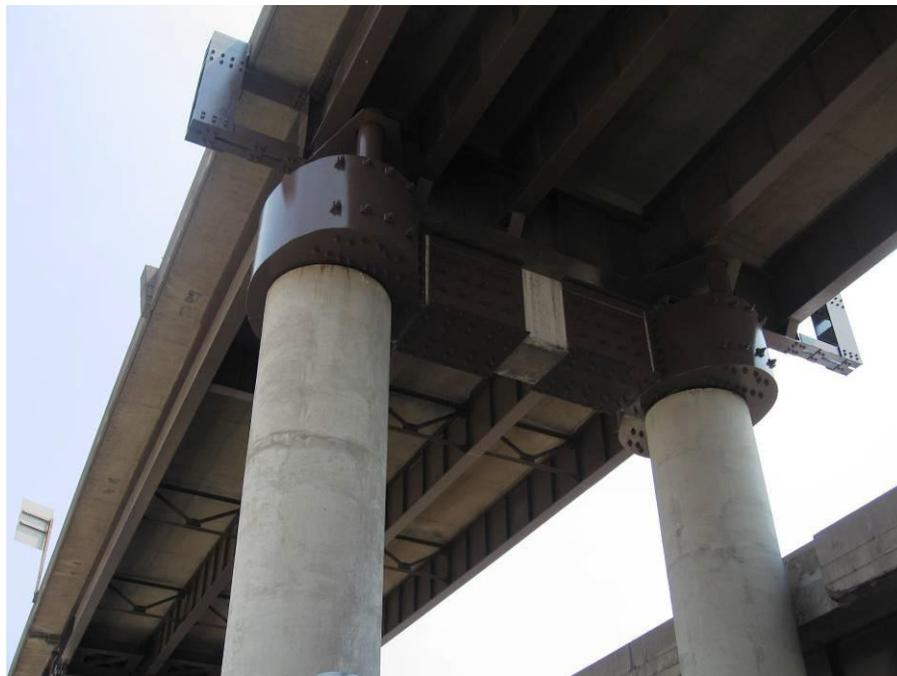
**Figure 95 Photo. Bent cap retrofits with reinforced steel encasement**
