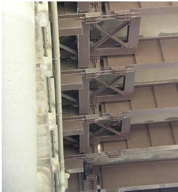
**Figure 189 Photo. Seat Extender and Restrainer Rods in Missouri: Seat Extenders (Poplar Street Complex – MO)**
