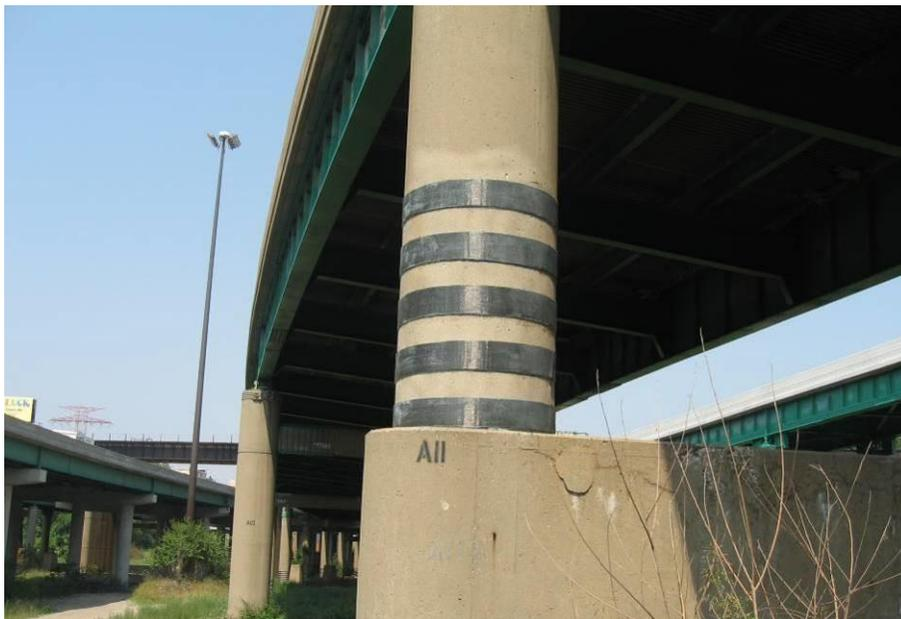
**Figure 169 Photo. Column Retrofits in Illinois: Fiber Composite Retrofit (Poplar Street Complex – IL)**
