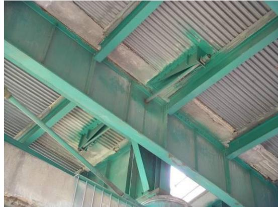
Figure 80 Photo. Connection details for high strength restrainer bars.
