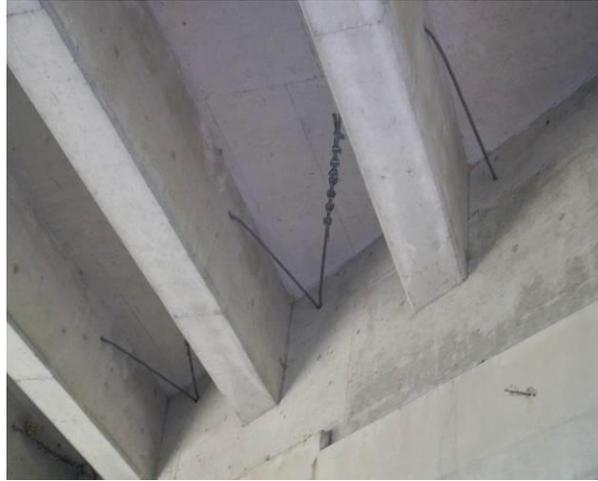
**Figure 174 Photo. Different restrainer cable configurations in Kentucky: Restrainer Cables**
