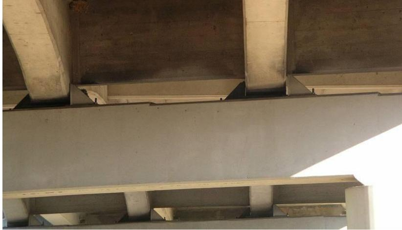
**Figure 212 Photo. Transverse Keeper Brackets (Shear Keys) in Tennessee: Keeper Brackets (Chambers Chapel Road over I40 – TN)**
