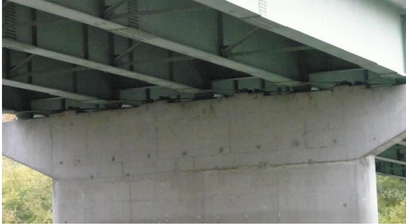
**Figure 150 Photo. Transverse restraining devices in Indiana: Transverse Restrainer Cables (SR51 over White River / Carl Grey Memorial Bridge – IN)**
