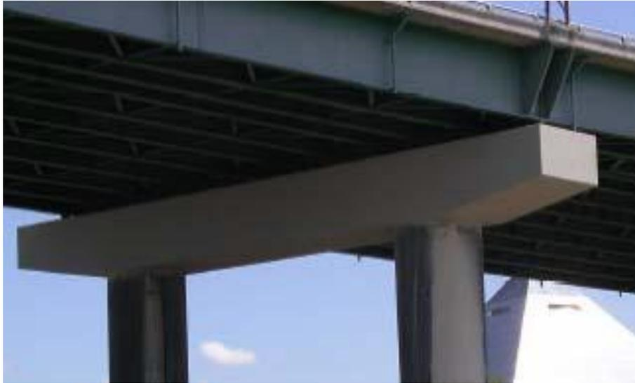
**Figure 94 Photo. Bent cap retrofits with reinforced concrete encasement.**
