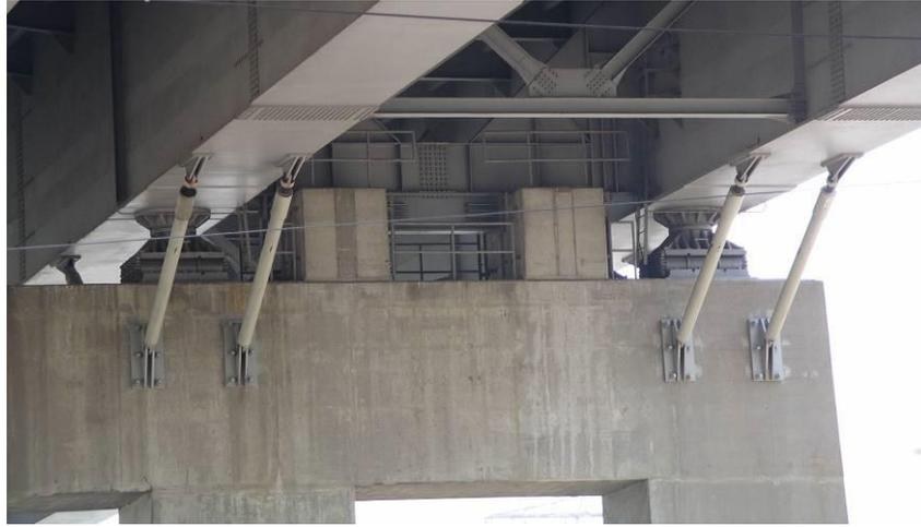
**Figure 175 Photo. Shear Key and Shock Transmission Unit Retrofits in Missouri:
