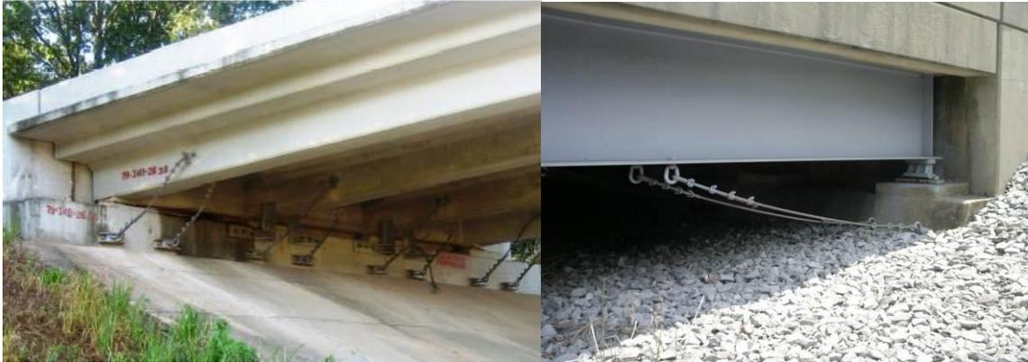
**Figure 76 Photo. Common CSUS restrainer cable retrofit details as performed in TN.**
