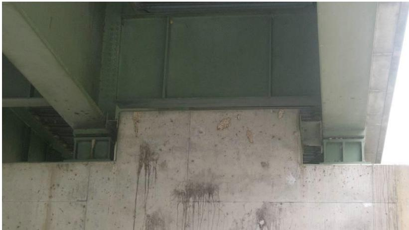
**Figure 149 Photo. Transverse restraining devices in Indiana: Transverse Shear Key (SR51 over White River / Carl Grey Memorial Bridge – IN)**
