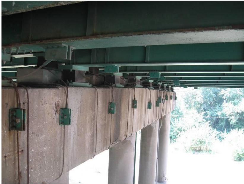
**Figure 170 Photo. Isolation in Illinois: Elastomeric Bearings and Restrainer Cables (Poplar Street Complex – IL)**
