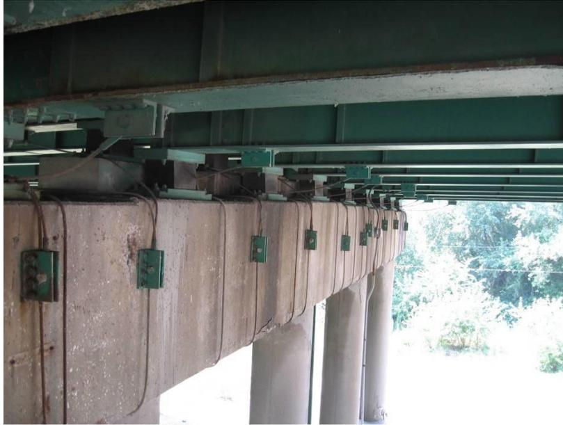
**Figure 78 Photo. Example of restrainer cables wrapped around bent cap.**
