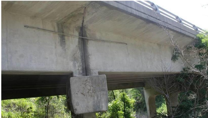
**Figure 173 Photo. Different restrainer cable configurations in Kentucky: Restrainer Cables**
