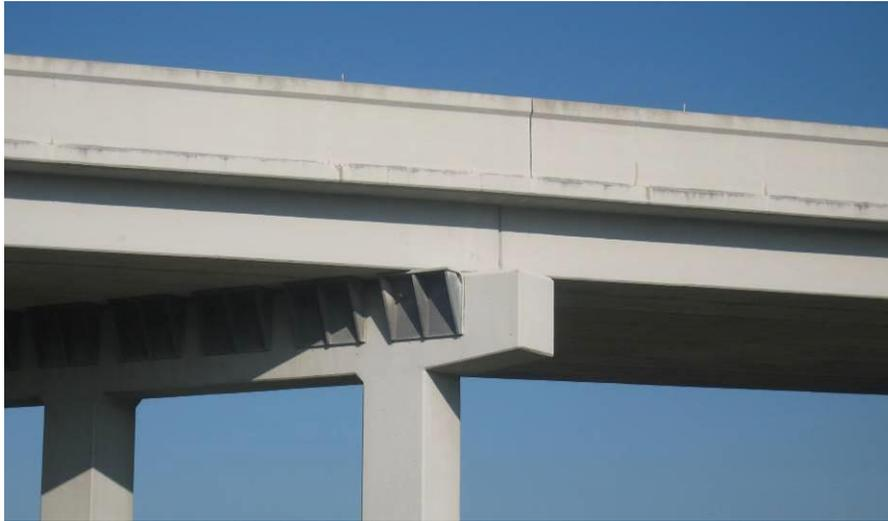
**Figure 224 Photo. Seat Extenders in Tennessee: Seat Extenders (RT A026 over I40 – TN)**
