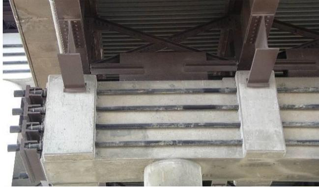
**Figure 181 Photo. Bumper, Bent Cap, and Shear Key Retrofits in Missouri: Bent Cap Post-tension Retrofit**
