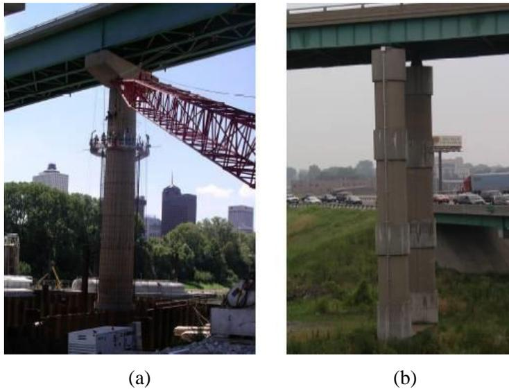
**Figure 64 Photo. Concrete column overlay (a) during construction in TN and (b) as a partial encasement in IL.**
