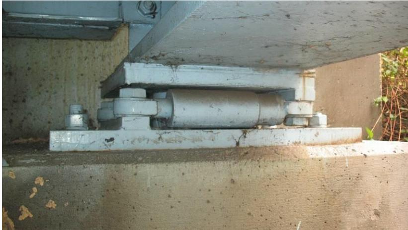
**Figure 148 Photo. Bearing retrofits and details in Indiana: Isomeric Bearing with Dampers (US 41 @ Eagle Creek –IN)**
