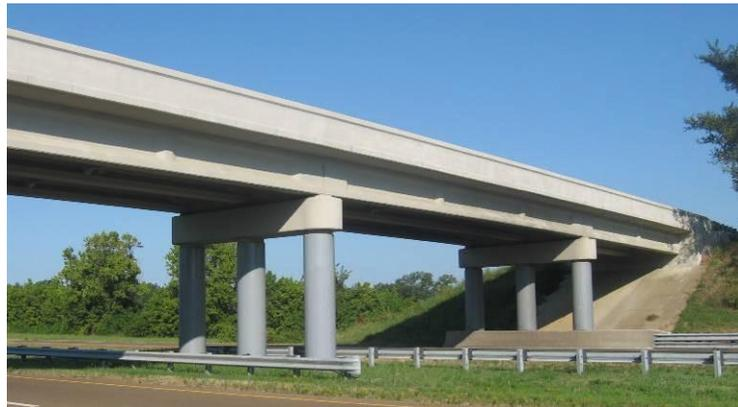
**Figure 204 Photo. Retrofit of Columns and Bent Caps in Tennessee: Steel Jackets and Bent Cap Retrofit (SR 196 over I40 – TN)**
