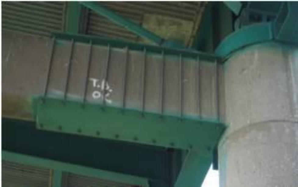
**Figure 93 Photo. Bent cap retrofit focused on shear reinforcement and confinement of the bent cap end regions.**
