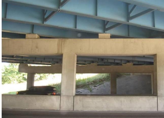
**Figure 203 Photo. Retrofit of Columns and Bearings in Tennessee: Bearing Retrofit (I40 over SR 15 – TN)**
