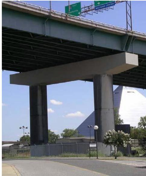
**Figure 226 Photo. Isolation and Column Retrofit of the Hernando DeSoto Bridge Carrying I40 between Tennessee and Arkansas: Reinforced Concrete Encasement with Steel Jackets (Hernando DeSoto I40 over Mississippi River - TN)**
