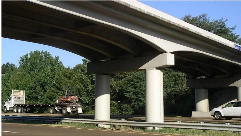
**Figure 214 Photo. Steel Jacket and Footing Retrofit in Tennessee: Steel Column Jackets (Chambers Chapel Road – TN)**
