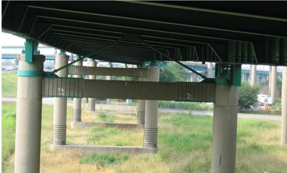
**Figure 152 Photo. Poplar Street Retrofits in Illinois: Column Cable Wraps, Bent Cap Retrofits, Transverse Restrainer Bars (Poplar Street Complex - IL)**
