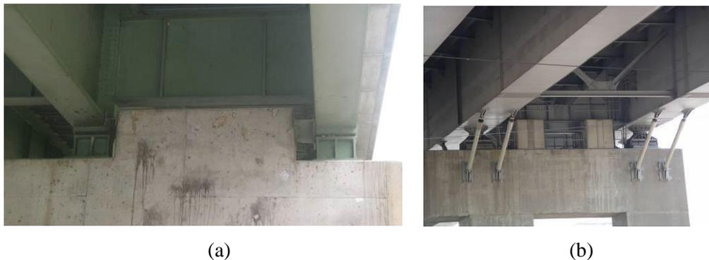
**Figure 85 Photo. Concrete block transverse shear keys in (a) Indiana (SR51 over White River/Carl Grey Memorial Bridge – IN) and (b) Missouri (Poplar Street Complex – MO).**
