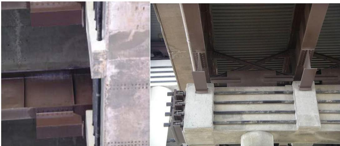
**Figure 82 Photo. Retrofits performed using bumper elements.**
