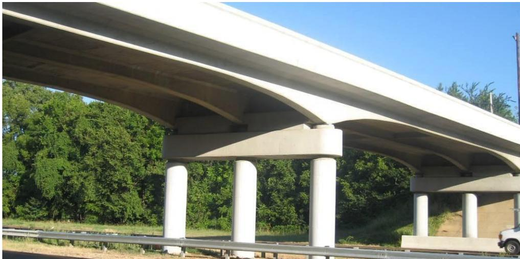
**Figure 198 Photo. Retrofit of Davies Plantation Road in Tennessee: Bent Cap Retrofit, Steel Jackets, and Shear Keys (Davies Plantation Road – TN)**
