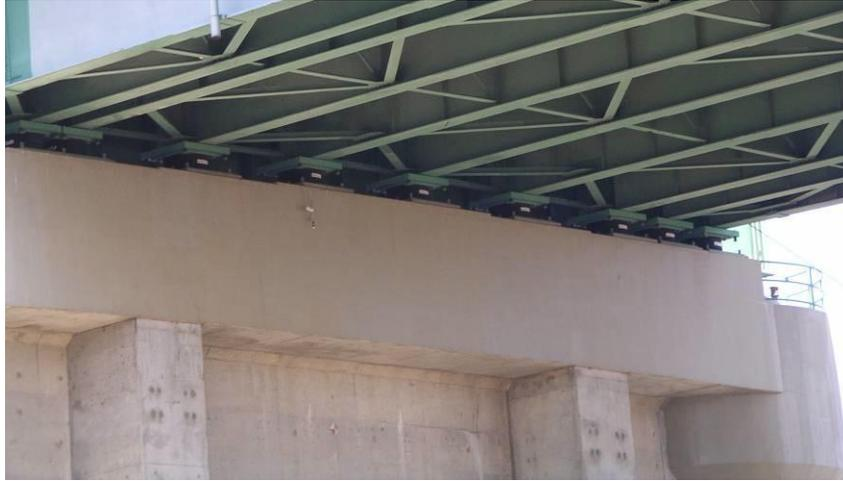
**Figure 228 Photo. Isolation and Column Retrofit of the Hernando DeSoto Bridge Carrying I40 between Tennessee and Arkansas: Elastomeric Isolation Bearings (Hernando DeSoto I40 Over Mississippi River – TN)**
