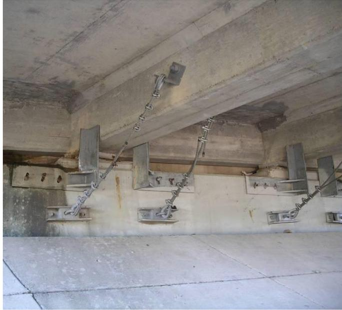
**Figure 207 Photo. Restrainer Cable Details in Tennessee: Restrainer Cables and Transverse Keeper Brackets (Chambers Chapel Road over I40 – TN)**
