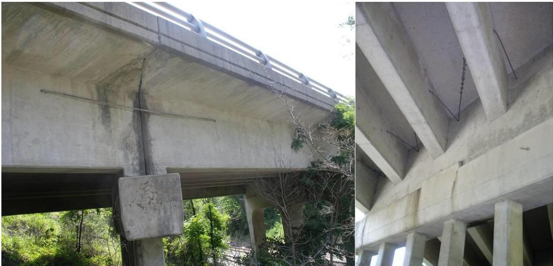
**Figure 77 Photo. Examples of restrainer cables connected between adjacent girders.**
