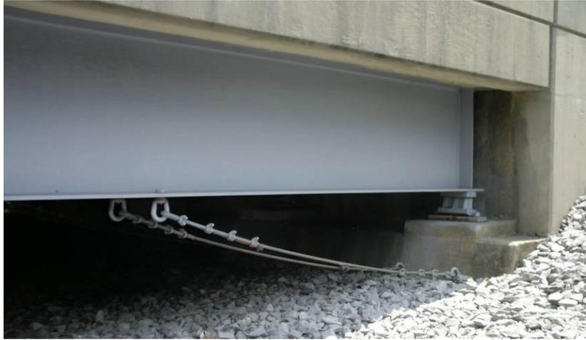
**Figure 172 Photo. Different restrainer cable configurations in Kentucky: Restrainer Cables**
