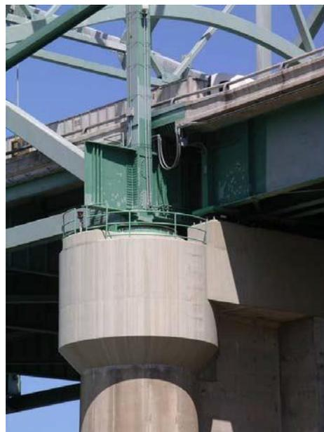
**Figure 227 Photo. Isolation and Column Retrofit of the Hernando DeSoto Bridge Carrying I40 between Tennessee and Arkansas: Friction Pendulum Isolation Bearing (Hernando DeSoto I40 Over Mississippi River – TN)**
