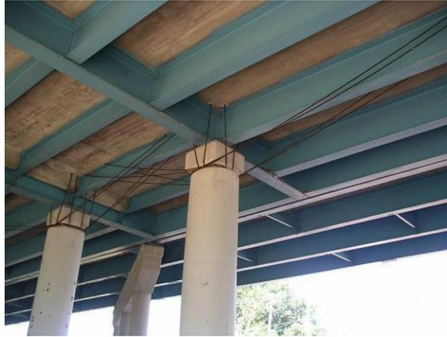
**Figure 193 Photo. The First Seismic Retrofit in Tennessee: First Retrofit in TN: “Uplift” and Longitudinal Restrainer Cables (SR 14 over CSX Railroad– TN)**
