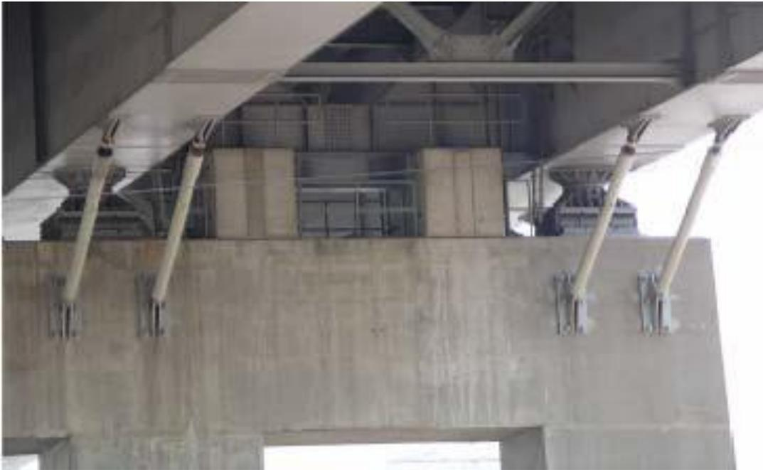
**Figure 83 Photo. Application of shock transmission units at the intermediate span of a bridge.**
