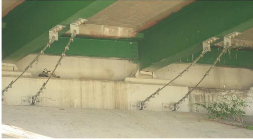
**Figure 221 Photo. Restrainer Cables in Tennessee: Restrainer Cables (SR59 – TN)**
