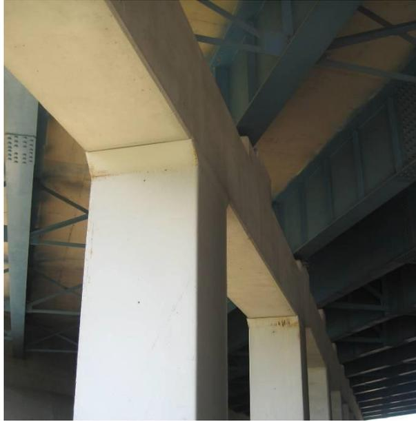
**Figure 201 Photo. Retrofit of Columns and Bearings in Tennessee: Painted Steel Jackets (I40 over SR 15 – TN)**
