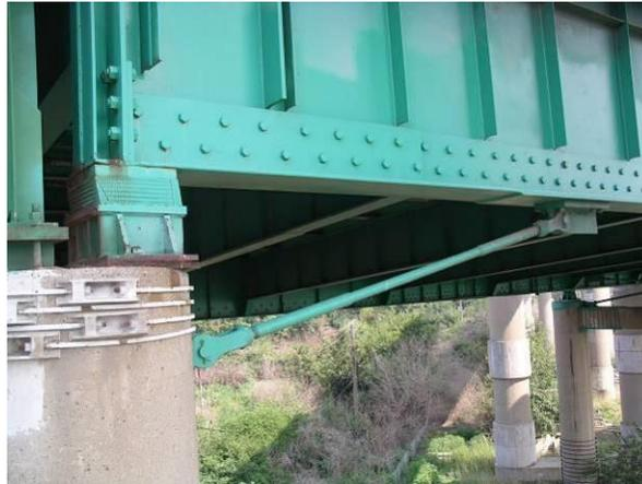
**Figure 160 Photo. Restrainer Bars and Bumpers in Illinois: Restrainer Bar (Poplar Street Complex - IL)**
