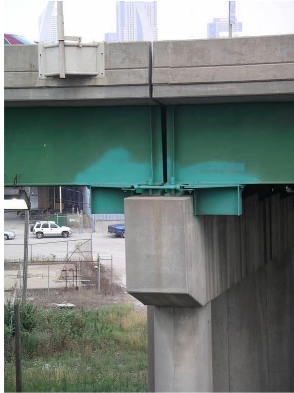
**Figure 162 Photo. Restrainer Bars and Bumpers in Illinois: Bumpers and Restrainer Bar (Poplar Street Complex - IL)**
