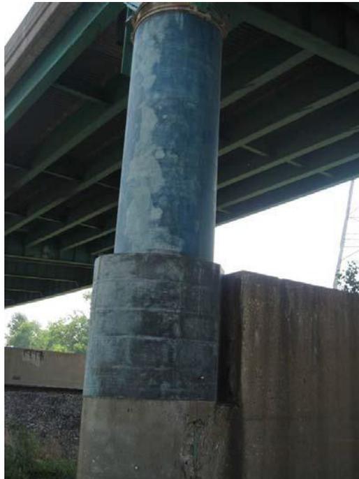
**Figure 167 Photo. Column Retrofits in Illinois: Fiber Composite Retrofit (Poplar Street Complex – IL)**
