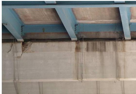
**Figure 194 Photo. The First Seismic Retrofit in Tennessee: First Retrofit in TN: “Deck Girder” Restraint Cables (SR 14 over CSX Railroad – TN)**
