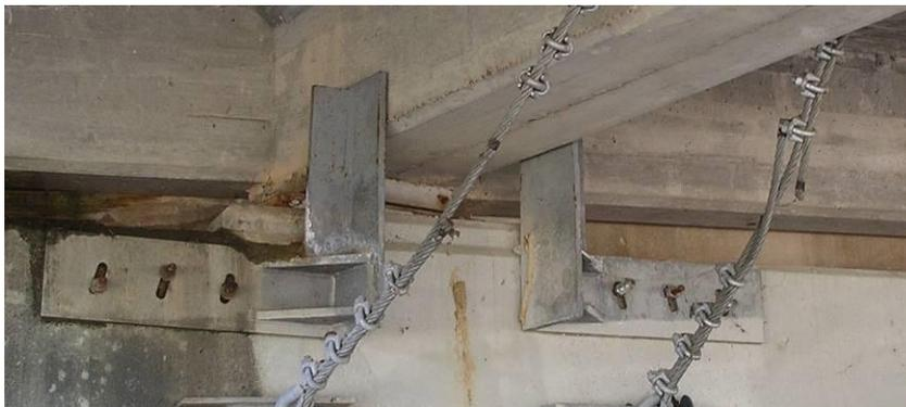
**Figure 210 Photo. Transverse Keeper Brackets (Shear Keys) in Tennessee: Transverse Keeper Brackets (Chambers Chapel Road over I40 – TN)**
