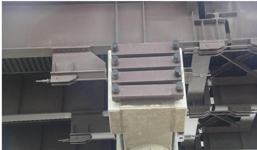
**Figure 182 Photo. Longitudinal Bumper and Restrainer Retrofits in Missouri: Restrainer Bars and Bumpers (Poplar Street Complex – MO)**
