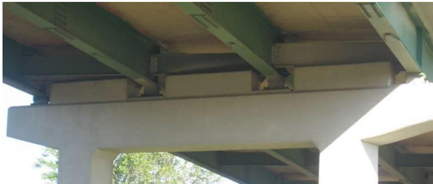
**Figure 217 Photo. Concrete Shear Keys in Tennessee: Concrete Shear Keys (SR59 over I40 – TN)**
