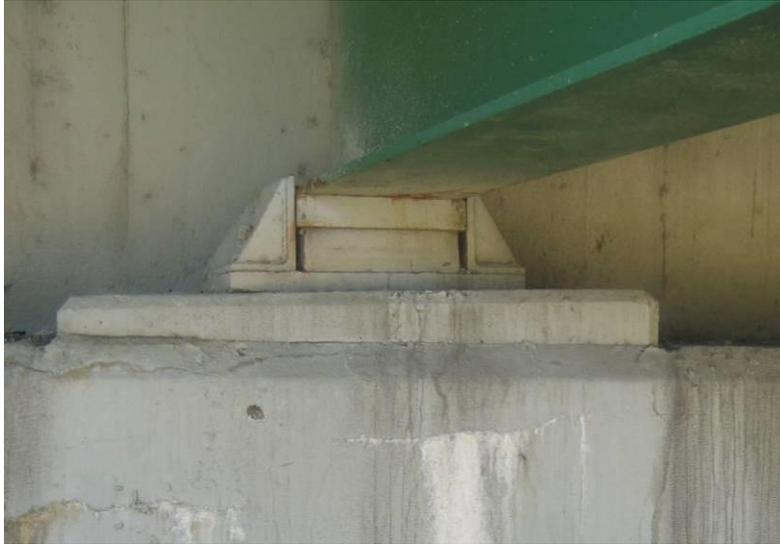
**Figure 219 Photo. Keeper Brackets in Tennessee: Keeper Brackets (SR59 – TN)**
