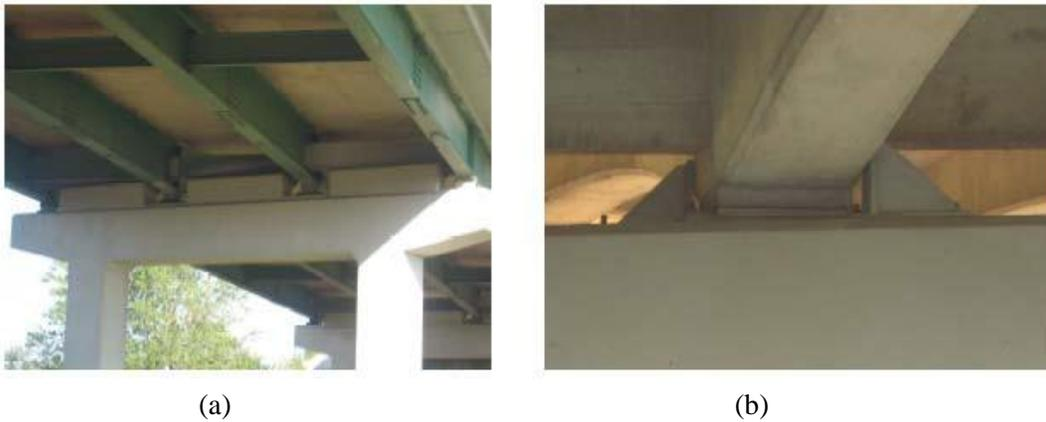
**Figure 84 Photo. Transverse restraint provided by (a) concrete shear keys and (b) keeper brackets.**
