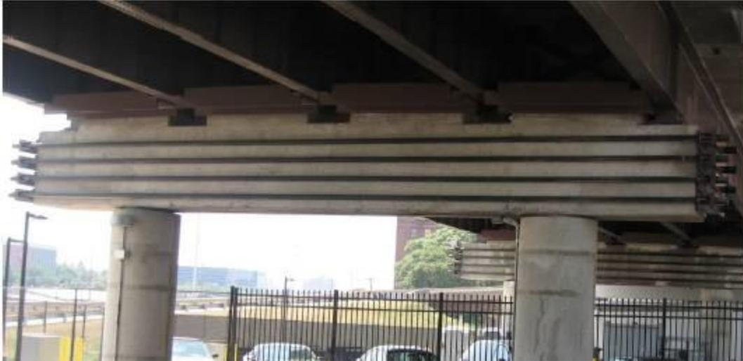
**Figure 92 Photo. Bent cap retrofit using post tensioning rods.**
