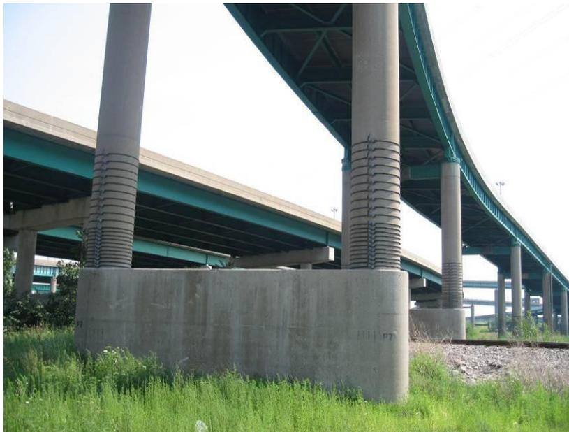
**Figure 157 Photo. Details of Column and Bent Cap Wraps in Illinois: Column Cable Wraps (Poplar Street Complex – IL)**
