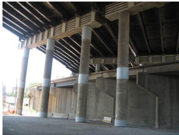
**Figure 184 Photo. Longitudinal Bumper and Restrainer Retrofits in Missouri: Steel Jackets (Poplar Street Complex – MO)**
