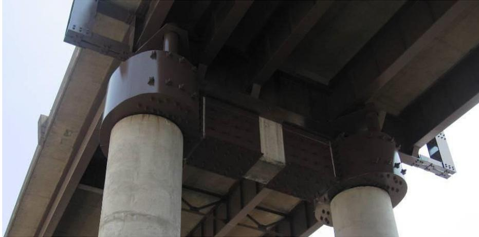
**Figure 188 Photo. Seat Extenders and Bent Cap Retrofit in Missouri: Bent Cap Retrofit (Poplar Street Complex– MO)**
