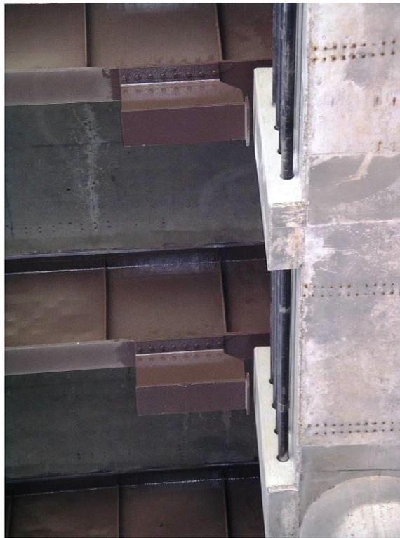
**Figure 178 Photo. Bumper, Bent Cap, and Shear Key Retrofits in Missouri: Bumpers (Poplar Street Complex – MO)**
