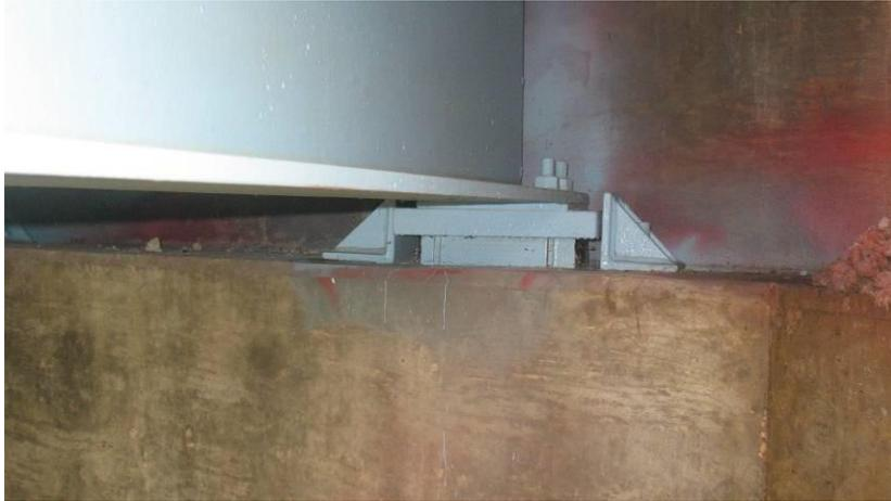
**Figure 146 Photo. Bearing retrofits and details in Indiana: Elastomeric bearing with keeper brackets (SR 66 at Diamond – IN)**
