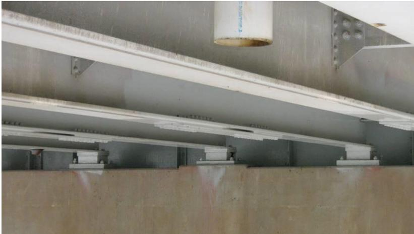
**Figure 147 Photo. Bearing retrofits and details in Indiana: Elastomeric Bearings (HW50 Red Skelton – IN)**
