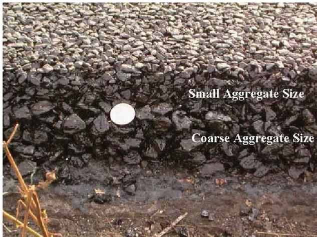
FIGURE 5-21 Example of a double-layer porous asphalt pavement used in the Netherlands. Source: Donovan (2006).
