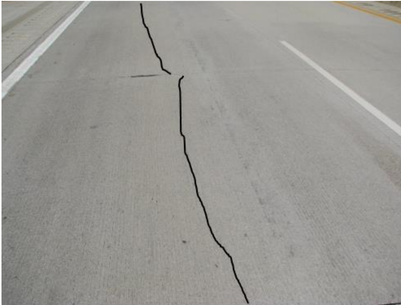
Longitudinal cracks on US 10 near Coleman (cracks digitally enhanced)
