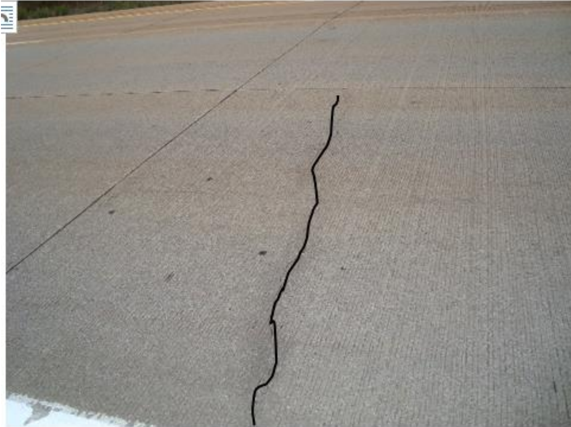
Longitudinal cracks on US 10 near Coleman (cracks digitally enhanced)
