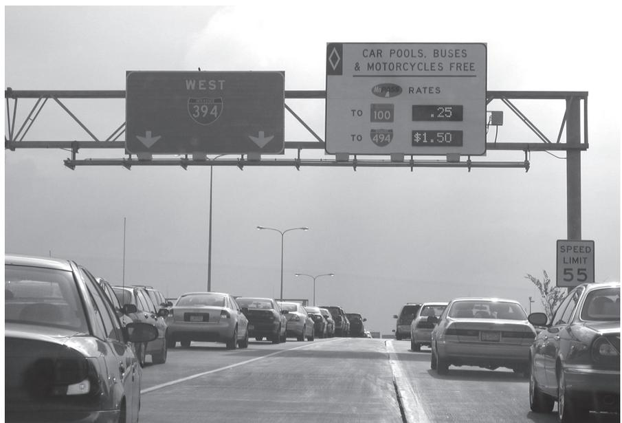
The MnPASS project, which uses dynamic pricing based on the level of congestion in the HOV lane, represents the first use of tolling in Minnesota and the first HOT project on concurrent flow HOV lanes. Photograph courtesy of the Minnesota Department of Transportation.
