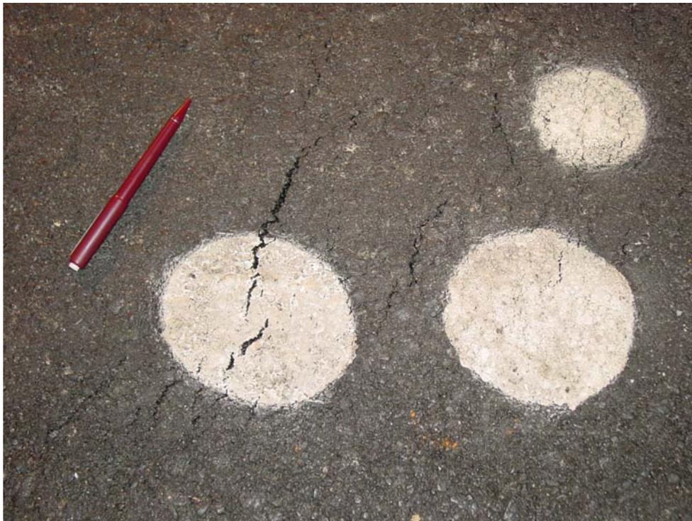
Figure 27. Close up of asphalt cracking over the emu sensors.
