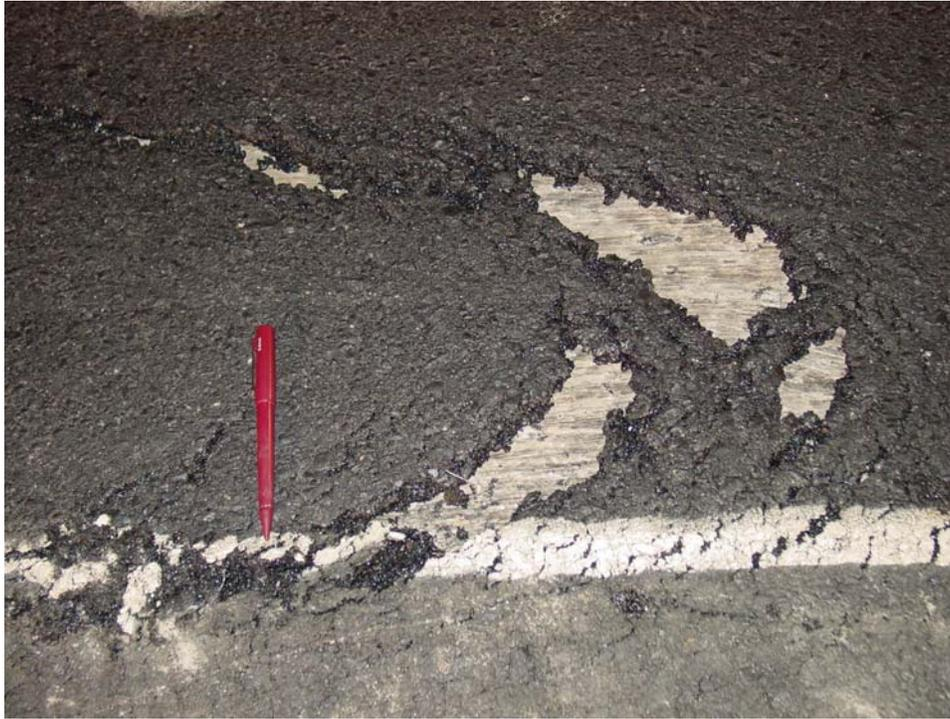
Figure 26. Close up of delaminated area showing striations on the lower asphalt layer.
